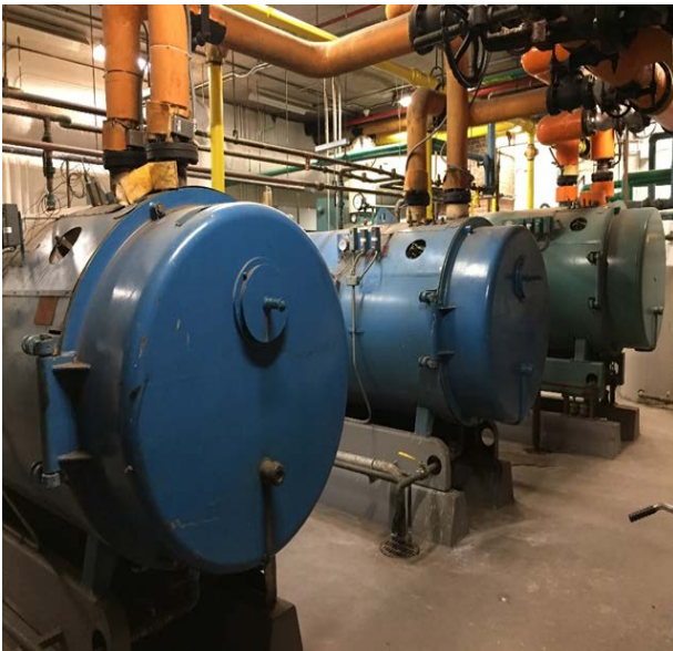
Cleaver Brooks Hot Water Boilers
