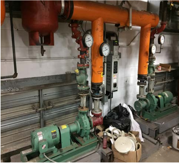
10 HP Hot Water Pumps and VFDs
