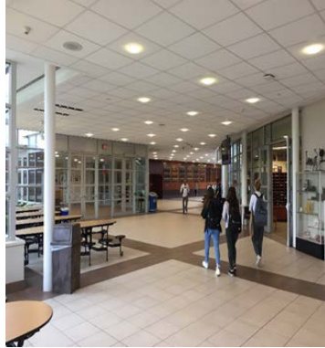
LED Tube, Atrium Recessed CFLs and Ceiling Mounted Occupancy Sensor
