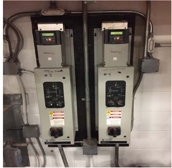
10 HP Hot Water Pumps and VFDs
