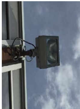
Wall Mounted CFL, Metal Halide Fixtures & a Timer
