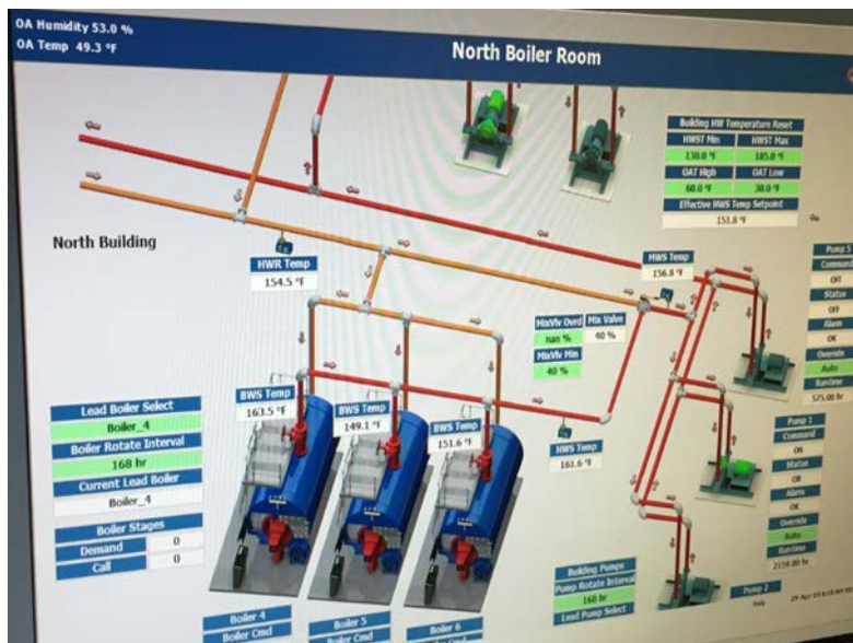
Steam Boilers EMS Control System
