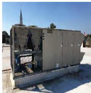
Image 12. Rooftop Packaged Unit
