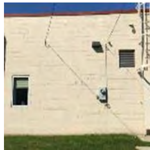
Image 3. Building Walls (Side)
