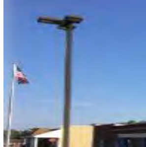
Image 10. Parking Lot Pole Fixtures
