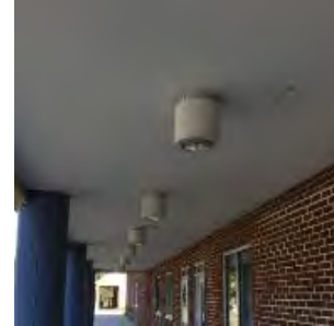
Image 11. Exterior Downlight Fixtures
