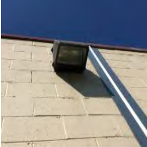
Image 9. Exterior Wall Pack
