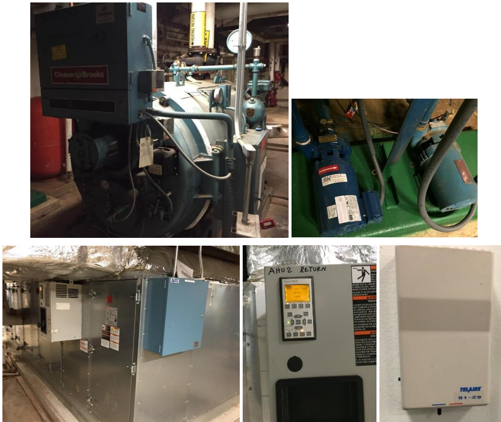
Image 3: HVAC Equipment - Boilers, Pumps, AHUs, VFDs, and Thermostats
