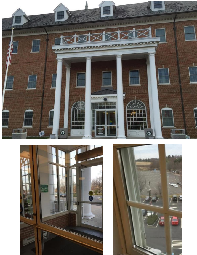
Image 1: Building Front Facade, Window and Door Frames
