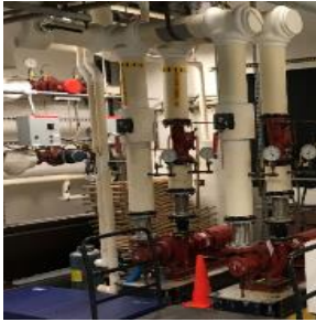
Heating Hot Water Pumps
