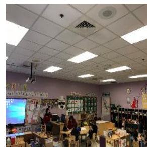
T8 Fixtures (Classroom)
