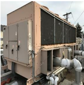
198-ton York Chiller
