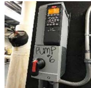
Chilled Water Pump VFD (P-6)
