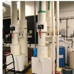
Chilled Water Pumps
