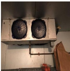
Walk-In Cooler (Evaporator)
