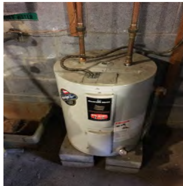
Domestic Hot Water Heater
