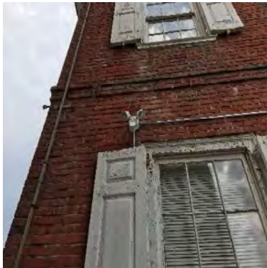
Exterior Flood Lights
