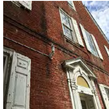
Exterior Porch Light
