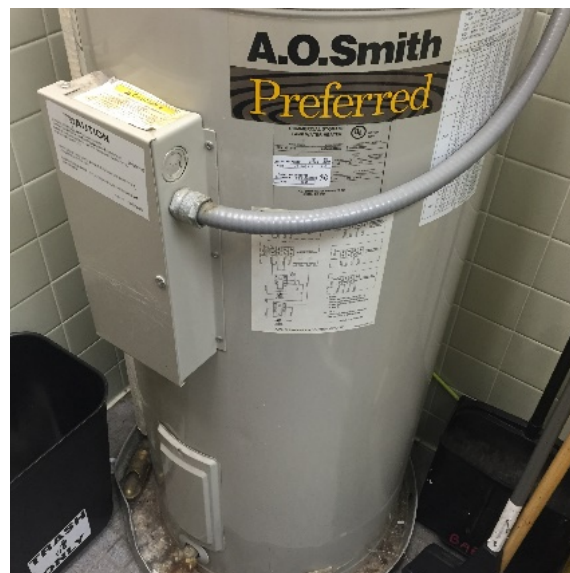
Figure 9 – Electric Hot Water Heater
