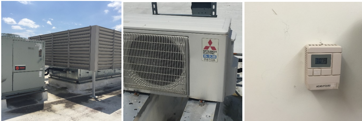
Figure 8 – Air Conditioning Equipment
