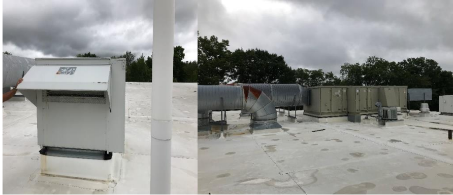
Image 6 Air Conditioning units and RTUs on roof
