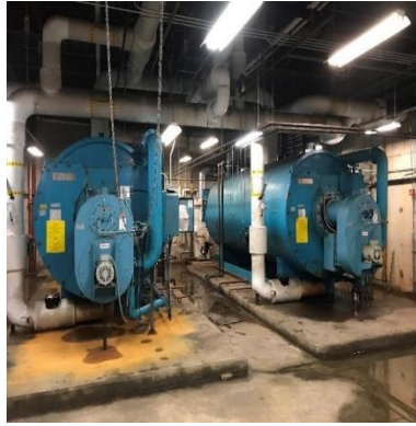
Image 4 Hot water boiler system
