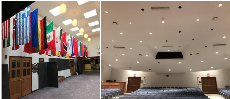
Image 2 School Interior Lighting
