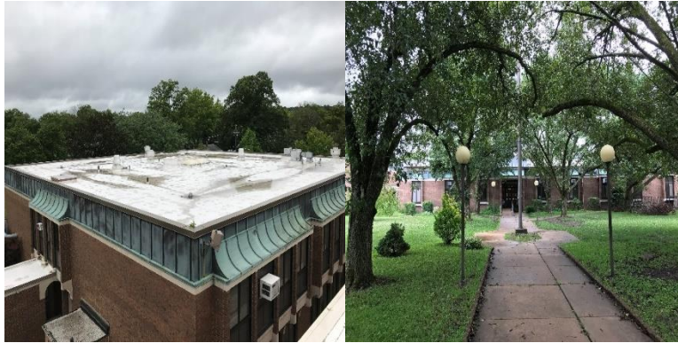
Image 1 Building Roof & Exterior
