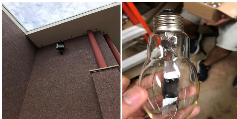
Image 3 School Exterior Lighting & sample lamp fixture
