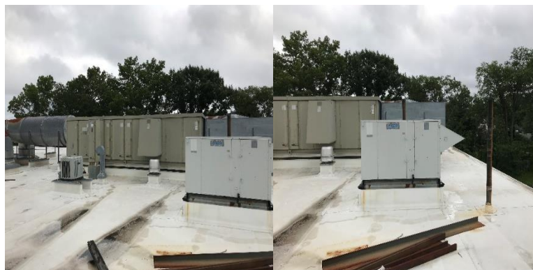
Image 5 Air handling units on roof
