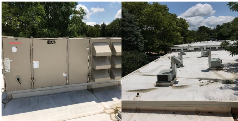
Image 5 Roof top units
