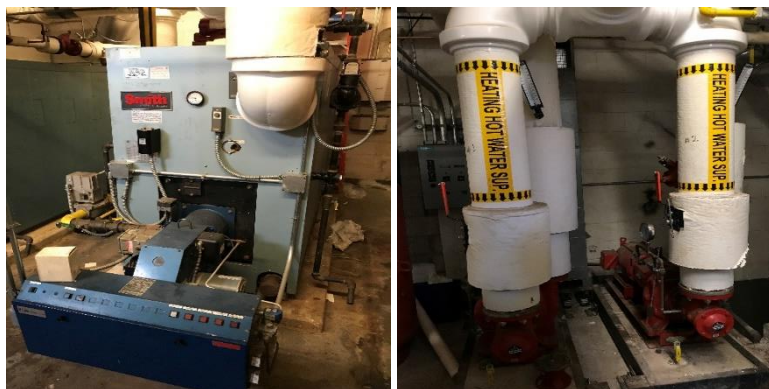
Image 4 Boiler system and hot water pumps
