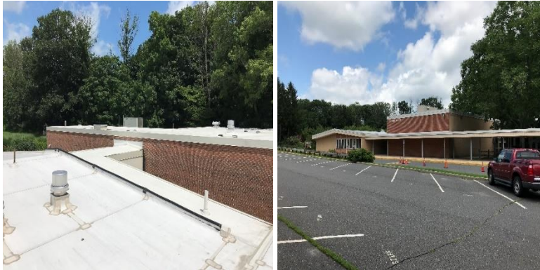
Image 1 Building roof and exterior
