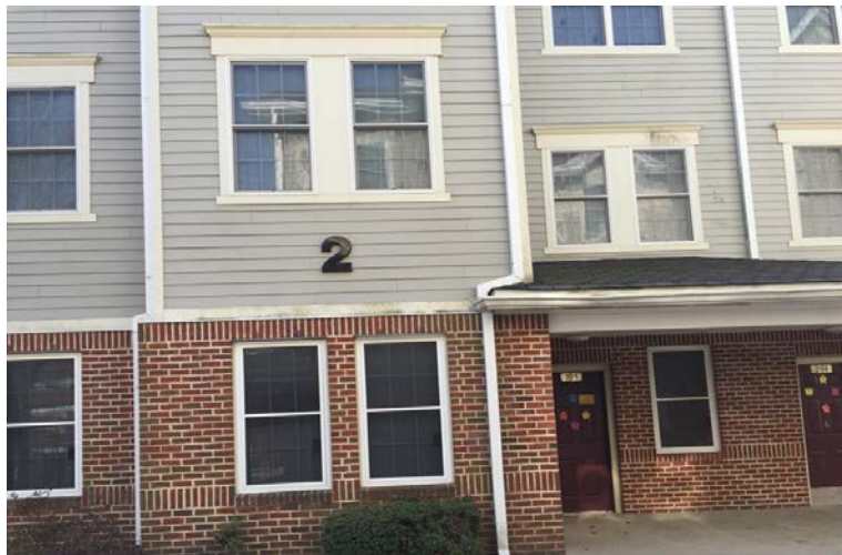
Image 1: Townhouse Windows and Doors
