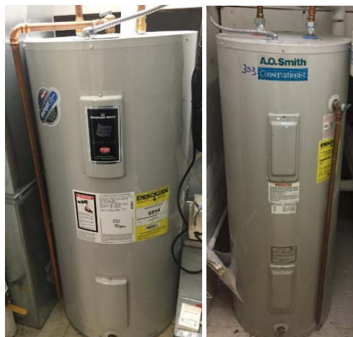
Image 7: Domestic Hot Water Heaters
