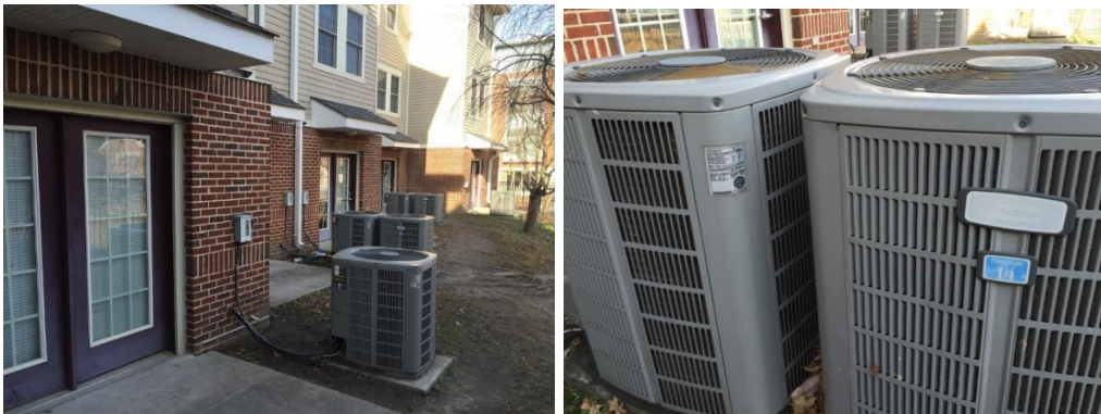
Image 4: Split System Condenser Units behind Each Townhouse
