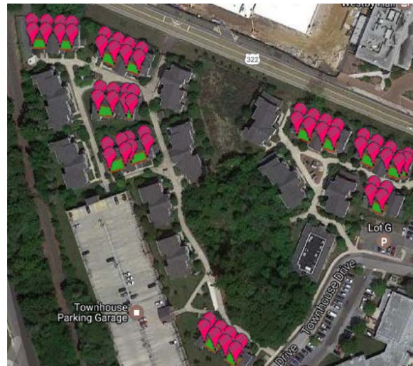
Image 11: Aerial View of Townhouse Complex
