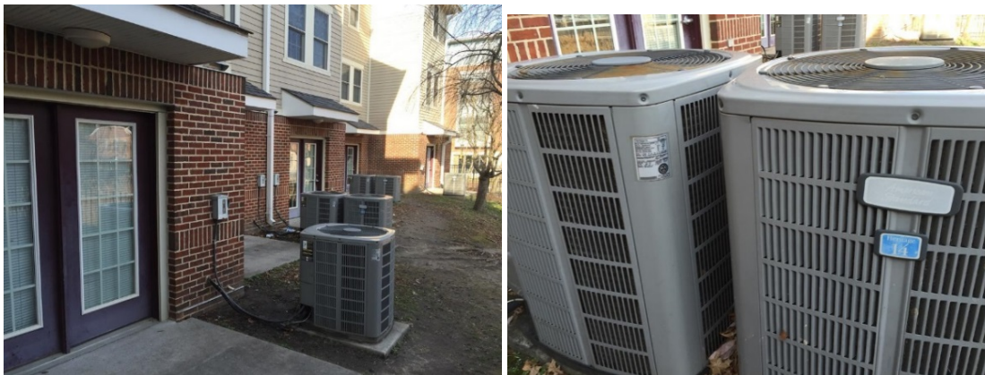
Image 4: Split System Condenser Units behind Each Townhouse
