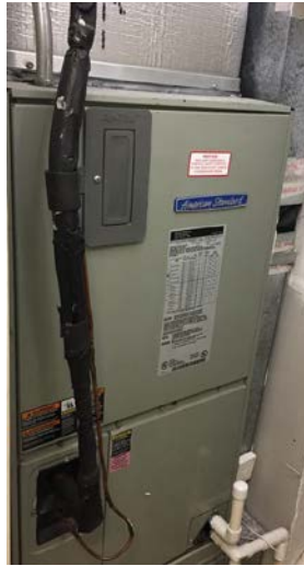
Image 6: AHU with electric resistance heating in utility closet
