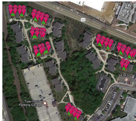
Image 11: Aerial View of Townhouse Complex
