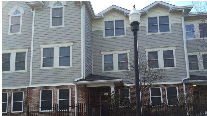
Image 1: Townhouse Windows and Doors
