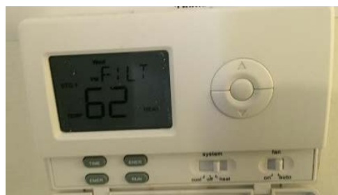
Image 5: Programmable Thermostats in Each Townhouse
