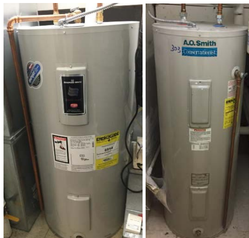
Image 7: Domestic Hot Water Heaters
