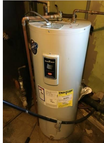
Annex Bldg - DHW
