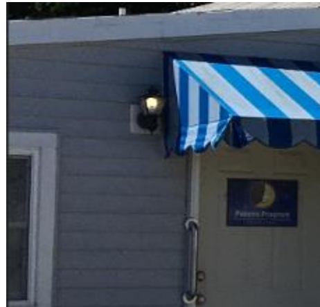
Annex Building– Entrance light (ON)
