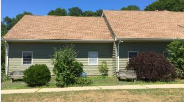
Nature Center siding, roof, windows
