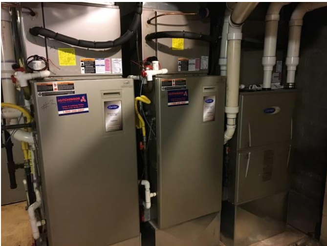
Nature Center – fan coil/furnace units
