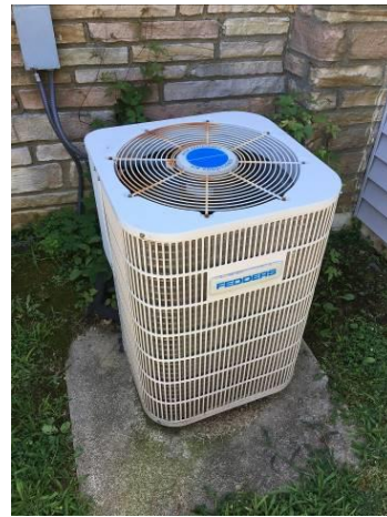
Annex Building – Condenser unit
