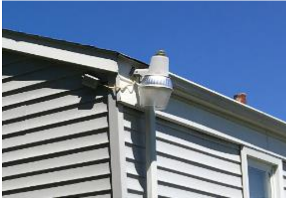
Annex Building– Metal Halide
