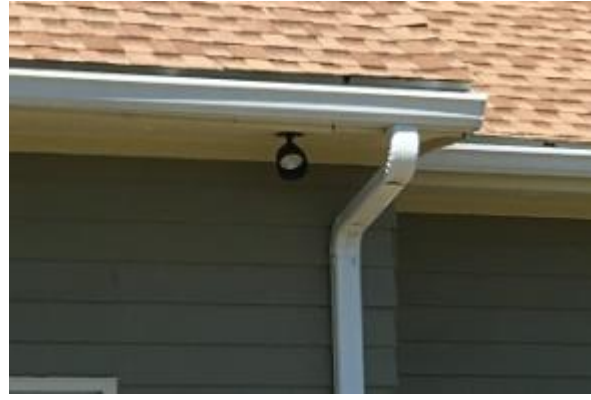
Nature Center – LED Flood Light
