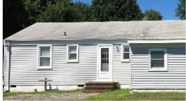
Annex Building siding, roof, windows, door
