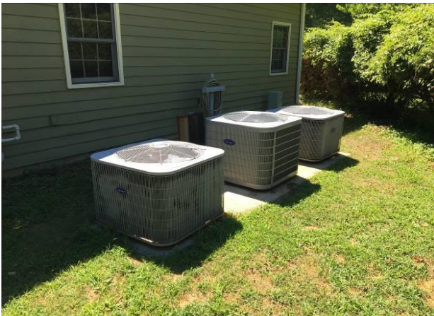
Nature Center – Condenser units
