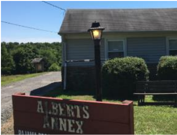
Annex Building– Pole light (ON)
