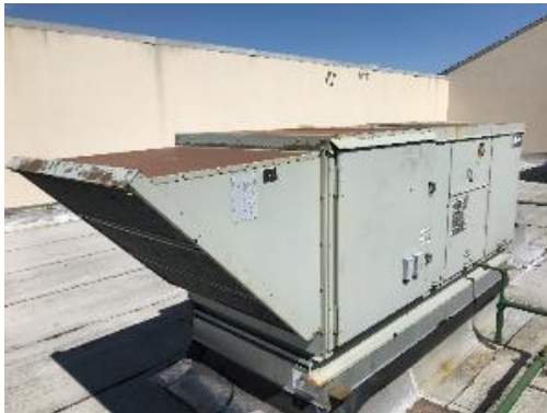
Roof top unit
