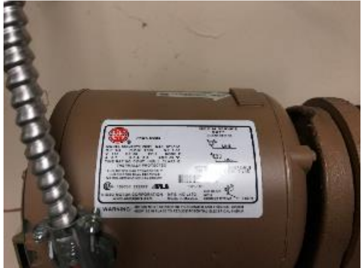
DHW circulation pump
