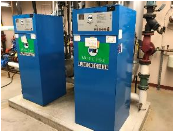
Hot water boilers
