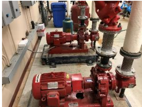
Heating hot water pumps
