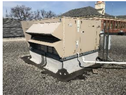
Roof top unit
