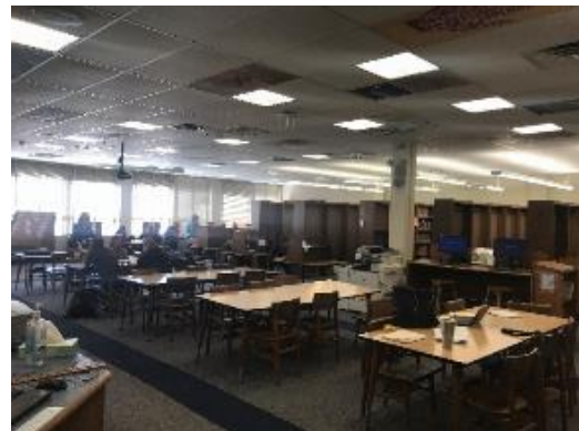
Media center lighting
