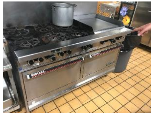
Gas stove with griddle
