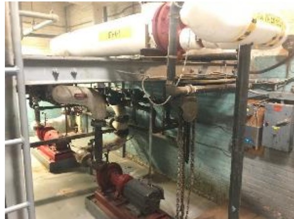
Heating hot water pumps
