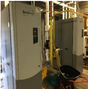
Aerco Benchmark 2.0 condensing boilers
