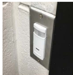
Wall mounted occupancy sensor
