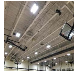
Gymnasium high-bay LED fixtures
