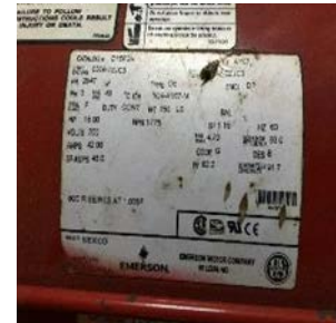
HHW pump motor nameplate
