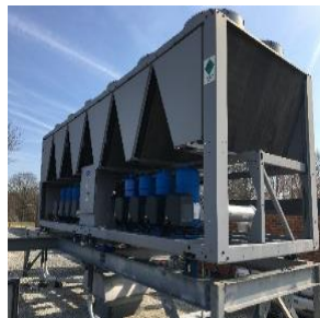
Carrier rotary scroll air-cooled chiller
