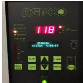
Aerco Benchmark 2.0 control panel
