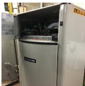
Domestic water heater
