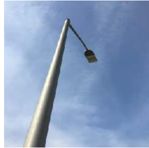
Pole mounted LED fixture
