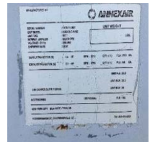
Multi-zone AHU nameplate
