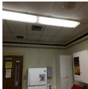
Typical surface mounted linear fluorescent fixtures
