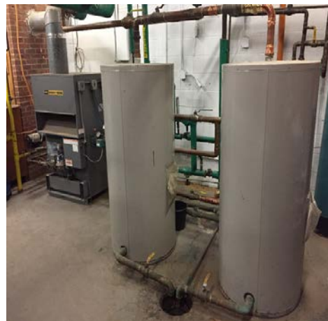
North Building and Kitchen Domestic Water Heater
