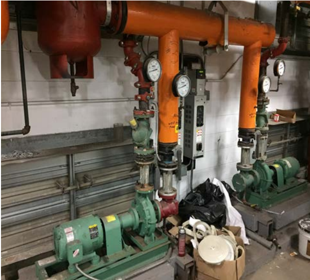
10 HP Hot Water Pumps and VFDs
