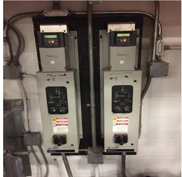
10 HP Hot Water Pumps and VFDs
