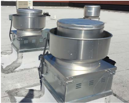
North & South Building Exhaust Fans
