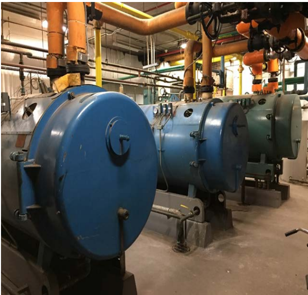
Cleaver Brooks Hot Water Boilers
