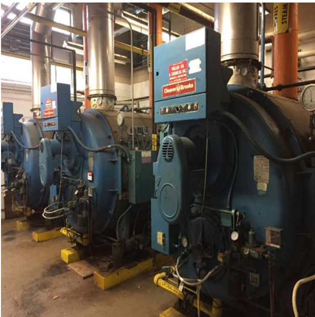
Cleaver Brooks Steam Boilers
