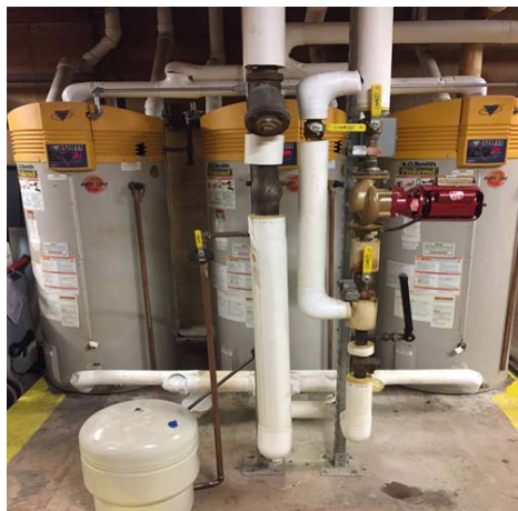
North Building and Kitchen Domestic Water Heater
