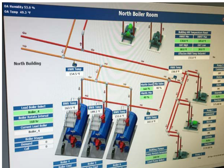
Steam Boilers EMS Control System
