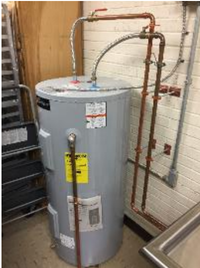
Electric Water Heater
