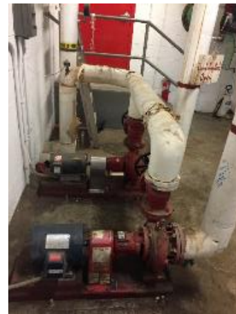
Heating Hot Water Pumps
