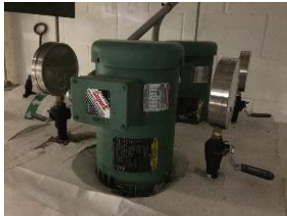
Chilled Water Pumps
