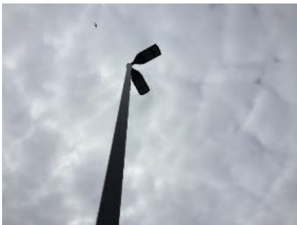
Exterior Pole Light
