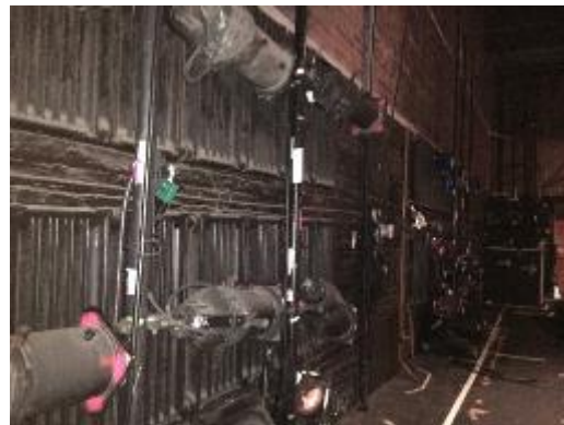
Hot Water Radiators on Stage
