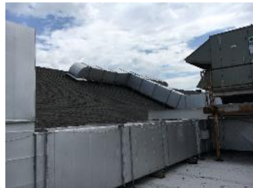
RTU – Back of House
