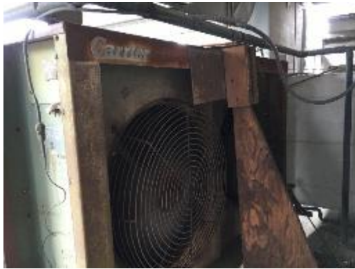
Outdoor Condensing Unit in Poor Condition
