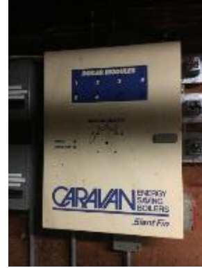
Lead Lag Controls in Boiler Room
