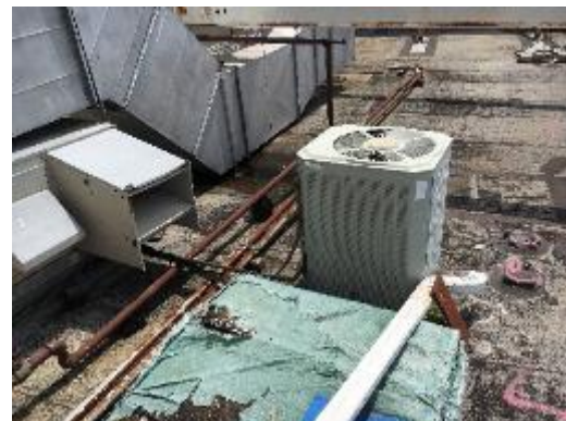
Outdoor Condensing Unit
