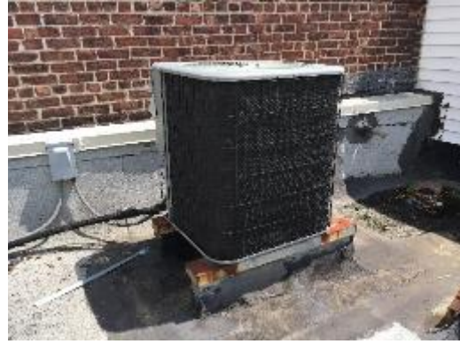
Outdoor Condensing Unit
