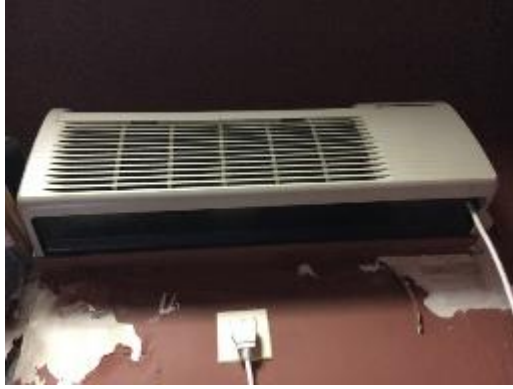
Ductless Split AC Indoor Unit
