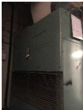
Indoor Unit – Admin Offices
