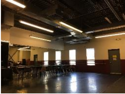
8-foot T12 Fixtures in Multipurpose Room
