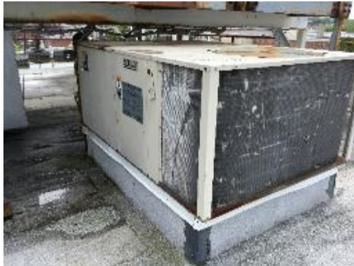
RTU – Building Addition
