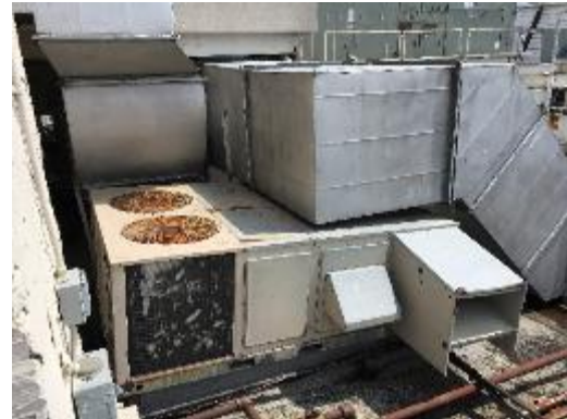
RTU – 2 nd & 3 rd Floor Building Addition
