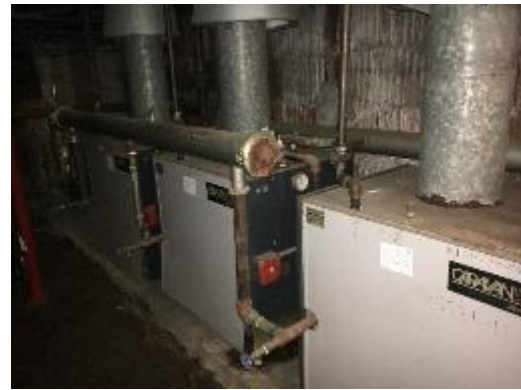
Hot Water Boilers
