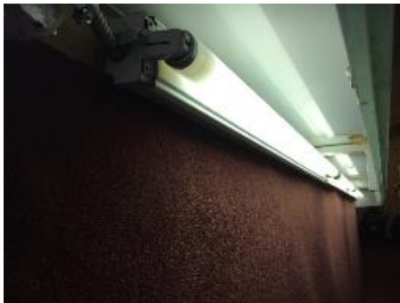
Under Bar T12 Lighting
