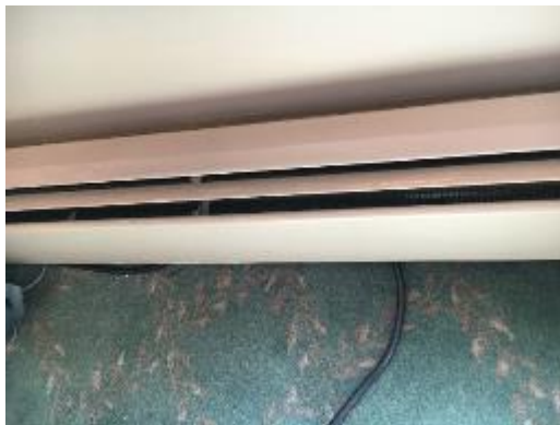
Hot Water Baseboard Heat in Offices
