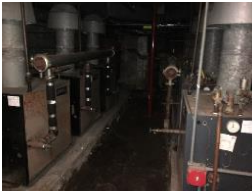
Hot Water Boilers
