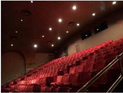
LED and Halogen Incandescent Fixtures in Theater
