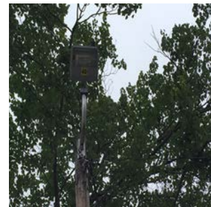
Exterior HID Fixture
