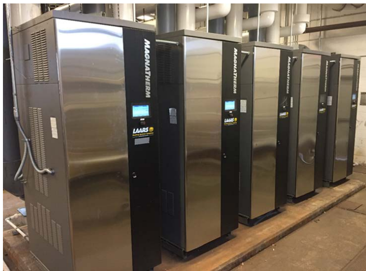
Condensing LAARS Boilers
