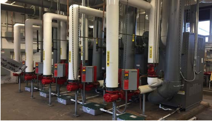
Hot Water Return Pumps and VFDs
