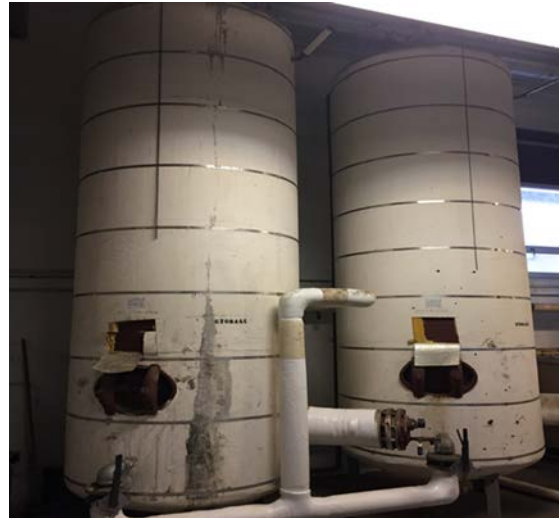
DHW and Storage Tanks
