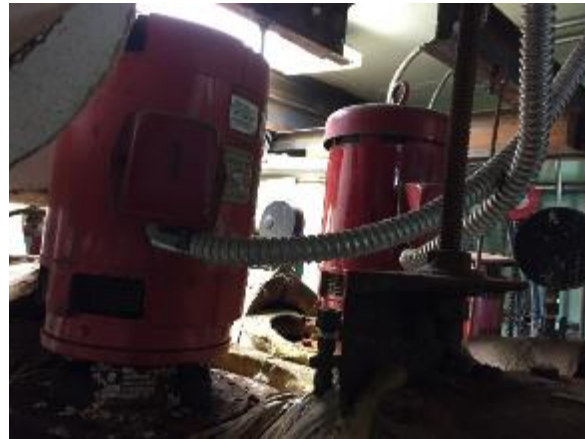
Heating Hot Water Pumps
