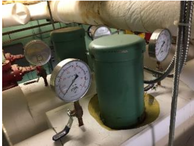
Chilled Water Pumps
