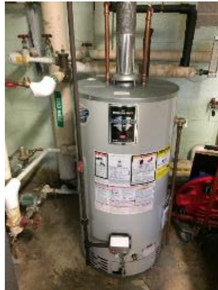
Gas Water Heater
