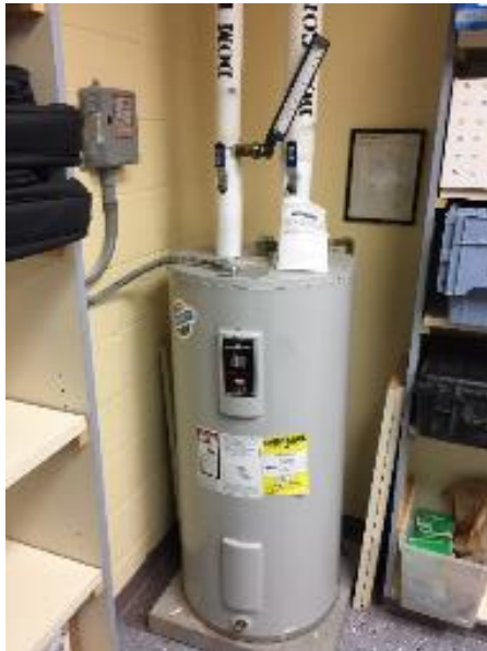
Electric Water Heater
