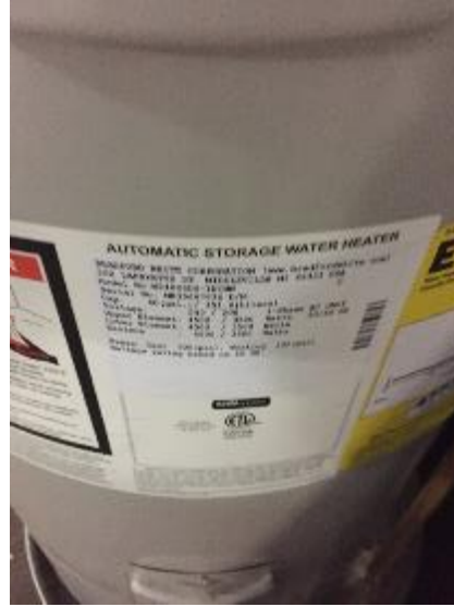
Water Heater Nameplate
