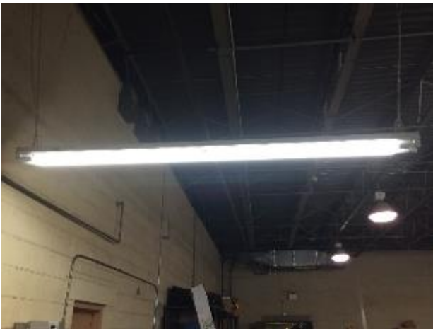
8 ft T12 Fixture
