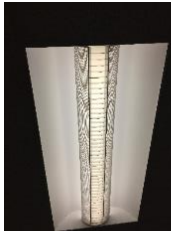
4 ft T8 Fixture
