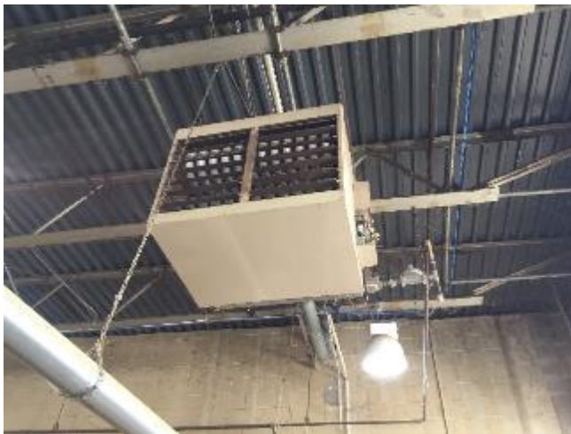
Warehouse Unit Heater
