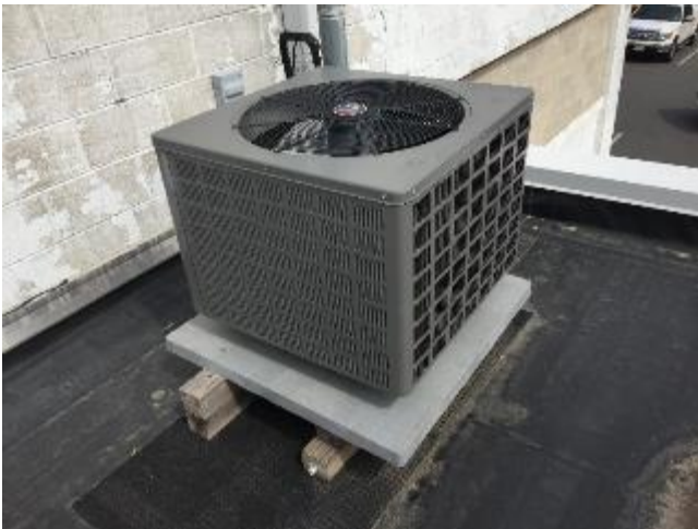
Split System on Lower Roof
