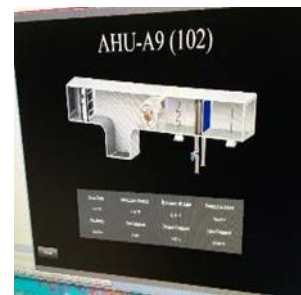
Delta Controls enteliWEB: AHU-9
