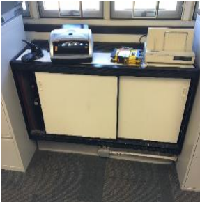
Main Office unit ventilator
