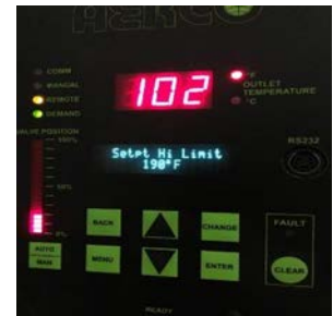
Benchmark 2.0 control panel showing high setpoint
