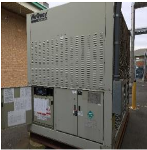
McQuay air-cooled chiller (PAC)
