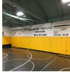
Wrestling room high-bay LED fixtures
