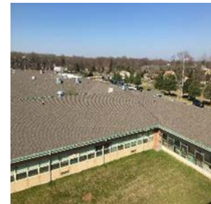
Pitched roof w/composite shingles
