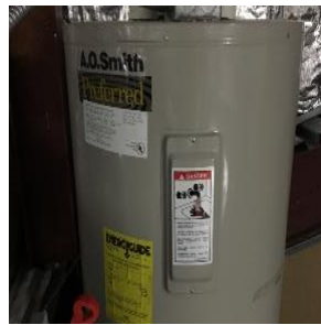
A.O. Smith 12 kW electric water heater (PAC)
