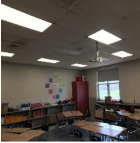
Common recessed T8 fixtures
