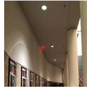
PAC LED recessed can lighting & LED exit signs
