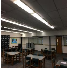
Typical surface mounted 2-lamp, 4-foot T8 fixture
