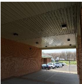
Typical canopy fixtures
