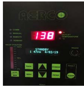
Aerco Innovation 1060 control panel
