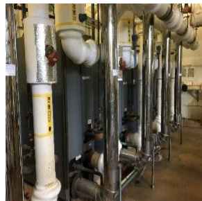
Backside of boilers and supply/return lines
