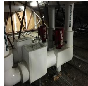
Secondary chilled water pumps (Daikin)
