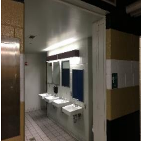
Boys locker room sinks
