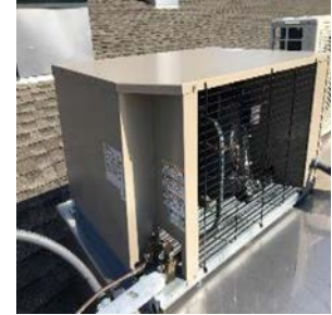
Walk in freezer condensing unit
