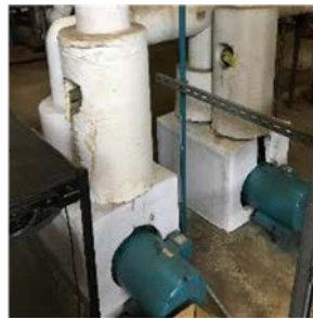
PAC chilled water pumps
