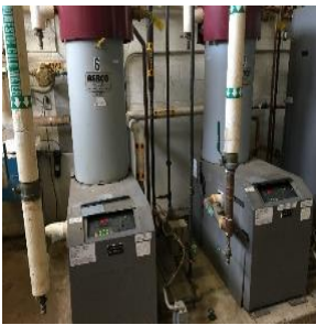
Aerco KC Series 1,000 MBh boilers
