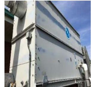
D Wing cooling tower for Heat Pump heat rejection
