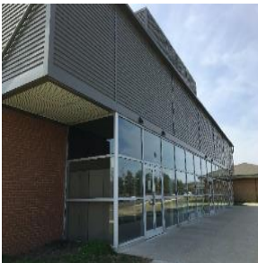
Brick exterior walls, aluminum framed windows and doors
