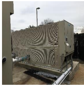
Daikin air-cooled chillers
