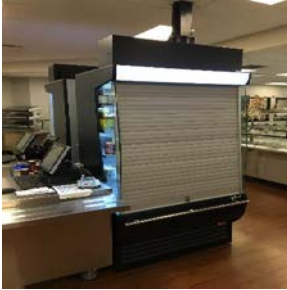
Refrigerated vertical open display cases
