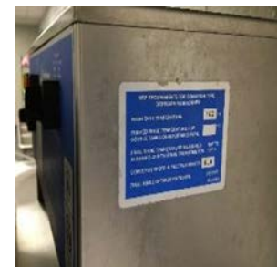
Dishwasher wash tank temp and belt speed
