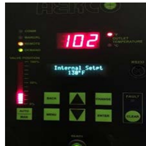
Benchmark 2.0 control panel showing current setpoint
