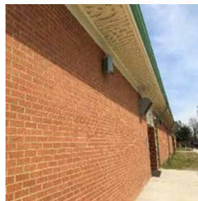
Metal Halide wall packs
