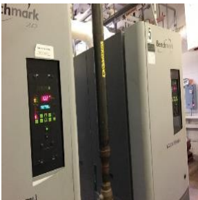
Aerco Benchmark 2.0 boilers
