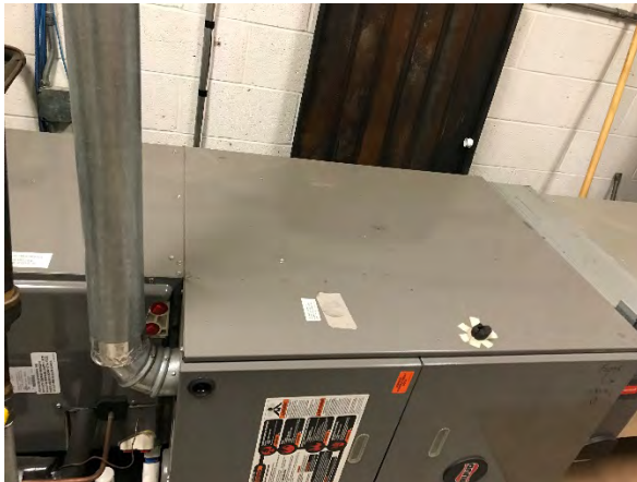
Packaged Cooling Coil
