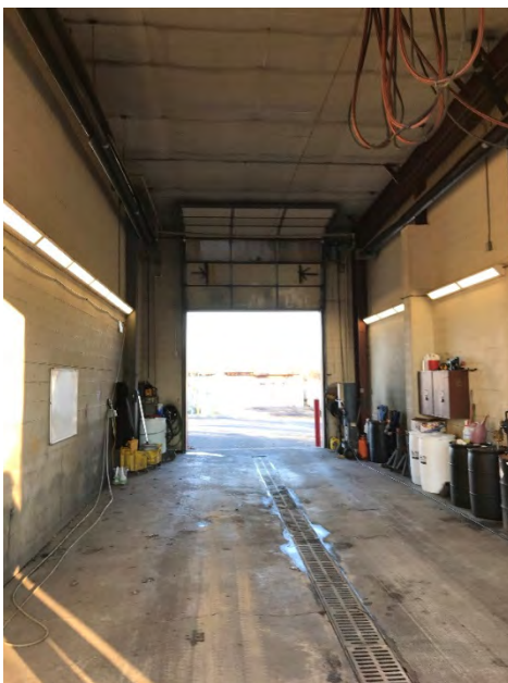
Wash Bay Lighting
