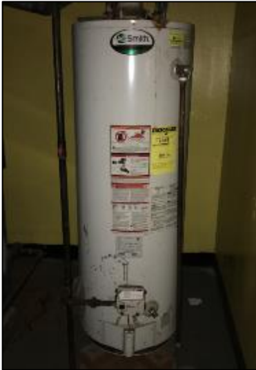
Operations Building DHW
