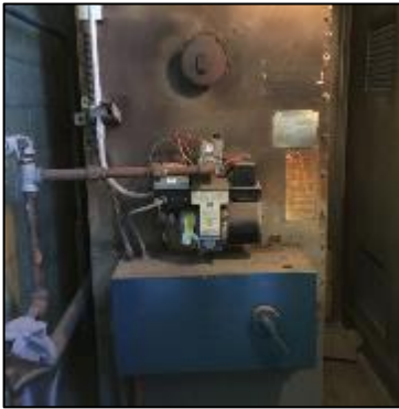
Grit Building Unit Heater
