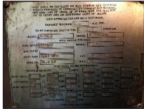
Grit Building Unit Heater
