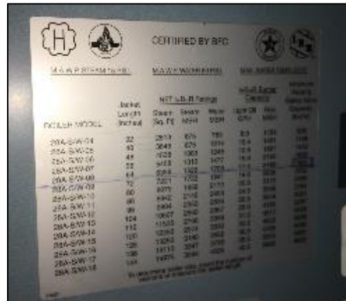
Operations Building Steam Boiler
