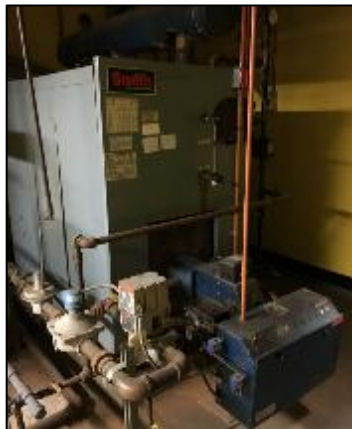
Operations Building Steam Boiler
