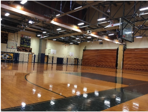
Linear Fluorescent T5HO lamp Fixtures in Gym
