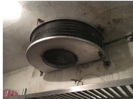
Walk-in Refrigeration Equipment, Evaporator
