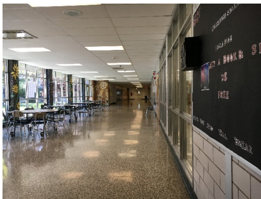
Linear Fluorescent T8 Recessed Troffer Fixtures
