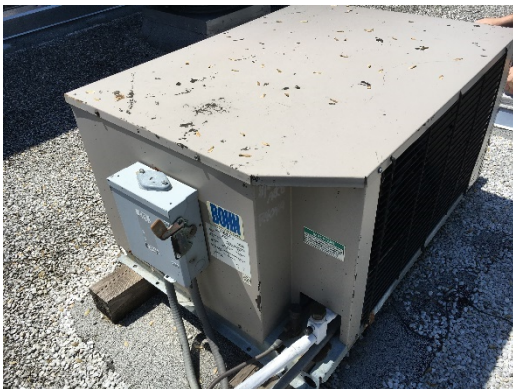
Walk-in Refrigeration Equipment, Compressors
