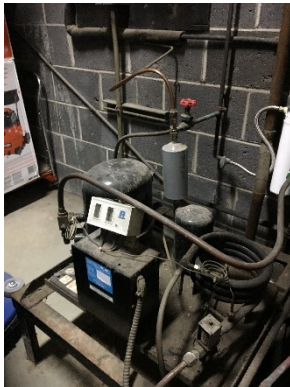
Walk-in Refrigeration Equipment, Compressor
