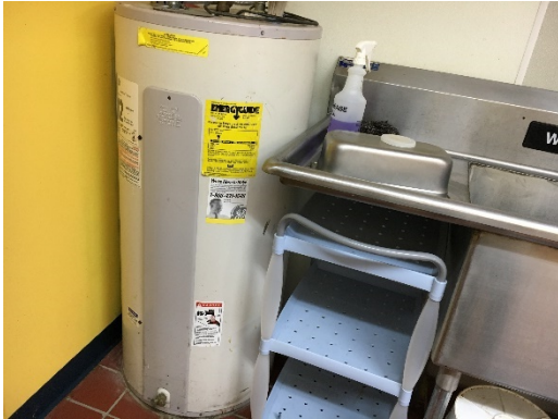
Snack Stand Electric Storage Tank Water Heater
