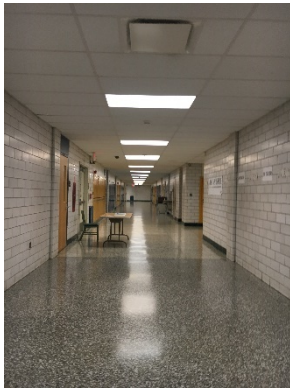
Linear Fluorescent T8 Recessed Troffer Fixtures
