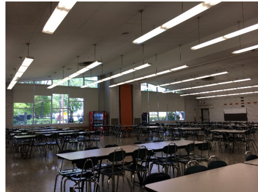
Linear Fluorescent T8 Pendant Mounted Continuous Row Wrap Fixtures
