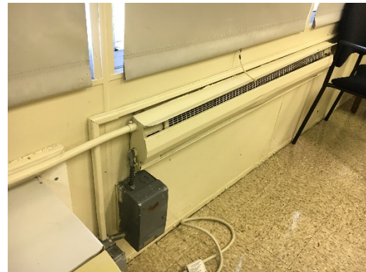
TC Building Electric Baseboard Heat
