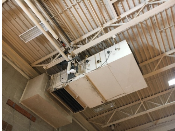
HV Unit in Auxiliary Gym
