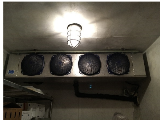
Walk-in Refrigeration Equipment, Evaporators
