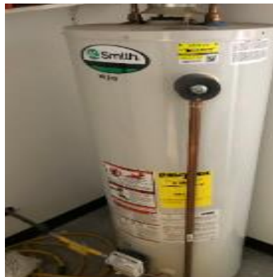
Domestic Hot Water Heater
