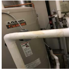
AO Smith Domestic Hot Water Heater
