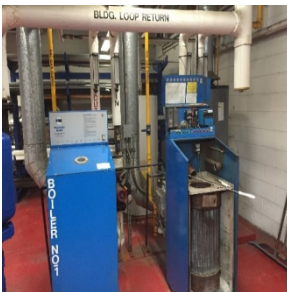
Hot Water Boilers
