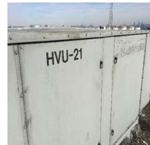
Heating and Ventilating Unit
