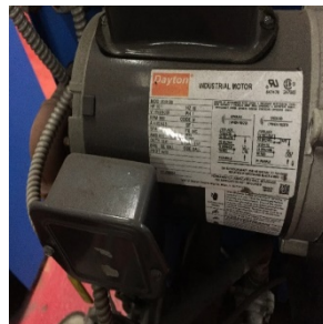
Heating Hot Water Pumps
