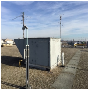
Packaged Rooftop AC Unit
