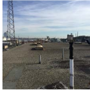
Roof with Gravel Finish
