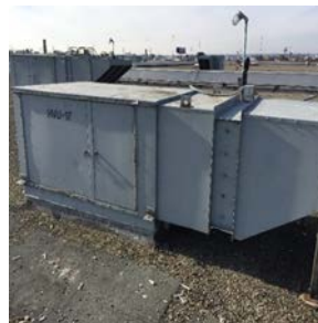
Heating and Ventilating Unit
