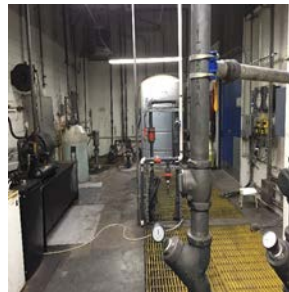
Bus Wash Area
