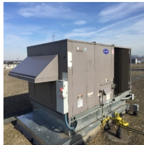
Packaged Rooftop AC Unit
