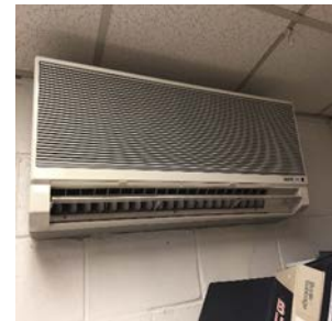
Split AC Unit
