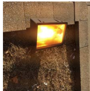
High pressure sodium Wall Packs
