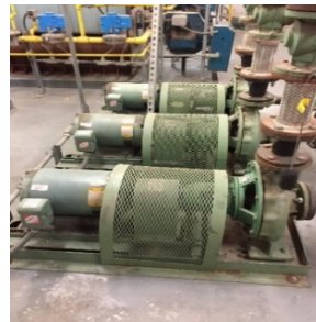
Hot water pumps
