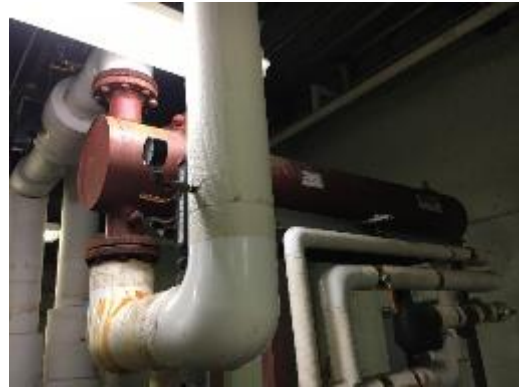
Shell and Tube Heat Exchanger
