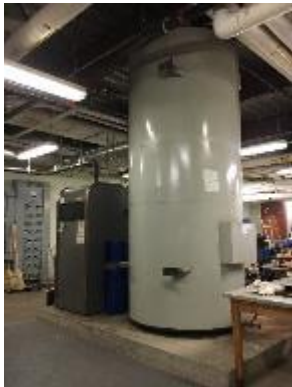
Domestic Hot Water Boiler and Storage Tank
