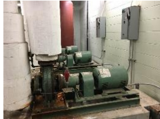
Chilled Water Pumps and Motors
