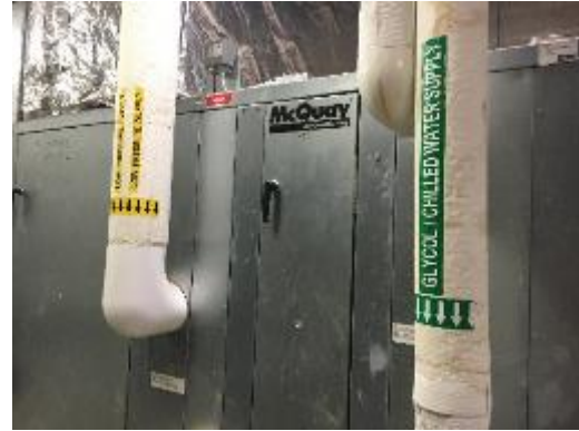
Air Handling Unit with Chilled Water and Steam Coils
