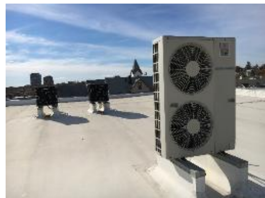
Outdoor Condensing Units for Split AC Systems
