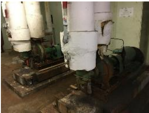
Hot Water Pumps and Motors
