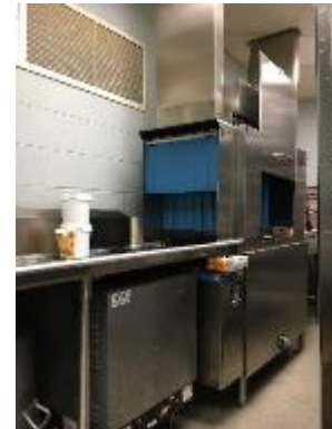
Dishwasher with Electric Booster Heater
