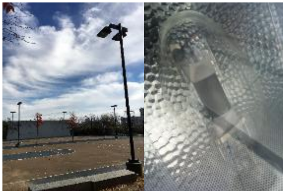
HID Pole Mounted and Flood Fixtures
