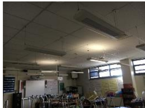
Linear T8 Pendant Mounted Fixtures
