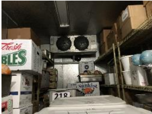
Indoor Evaporator Units for Walk-In Equipment
