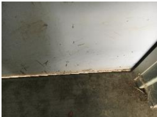
Exterior Door with Air Gap
