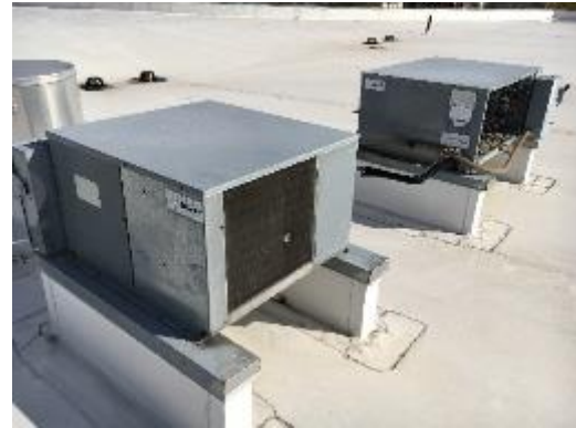
Outdoor Condensing Units for Walk-In Equipment
