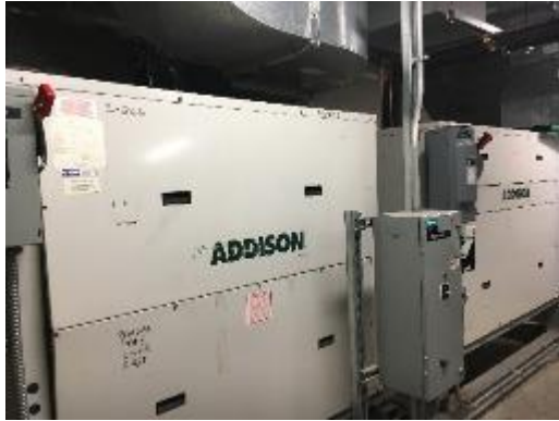
Air Cooled Condensing Units (ACCUs)
