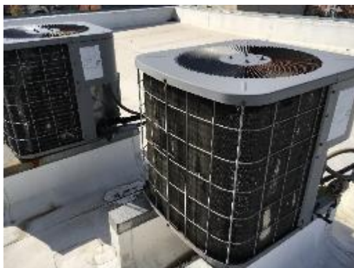
Outdoor Condensing Units for Split AC Systems
