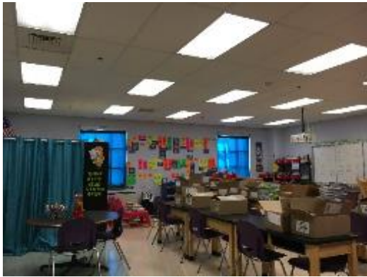
Linear T8 Recessed Troffer Fixtures
