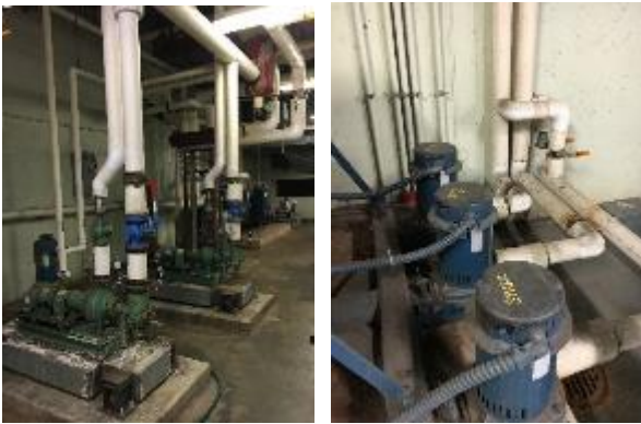
Boiler Feed and Condensate Return Pumps & Motors
