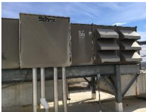
Roof Top Unit with Chilled Water Coil
