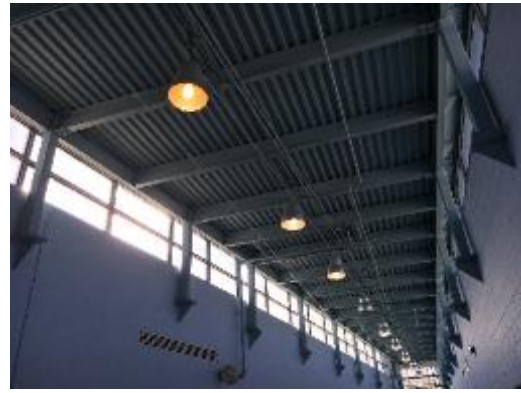
High Output Compact Fluorescent Lamp Fixtures
