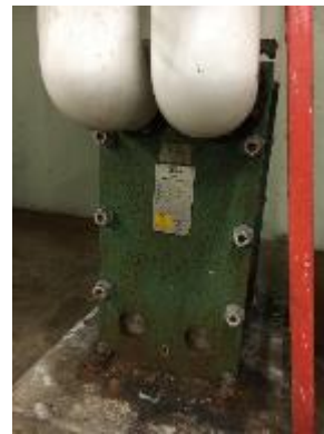
Plate and Frame Heat Exchanger
