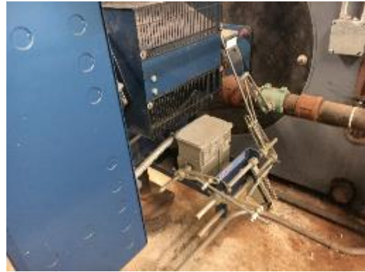
Mechanical Linkage Boiler Burner Controls
