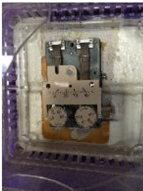
Manual Dial Thermostat in Poor Condition
