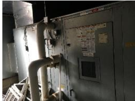
AHU serving the Cafeteria
