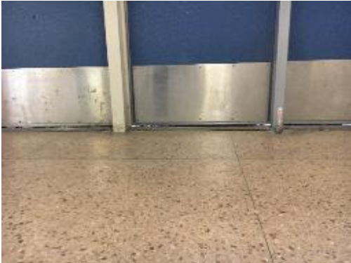
Weather-stripping in Poor Condition
