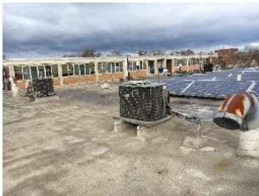
Outdoor Condensing Units for Split AC Systems
