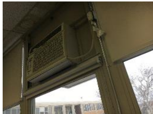
Window AC Unit
