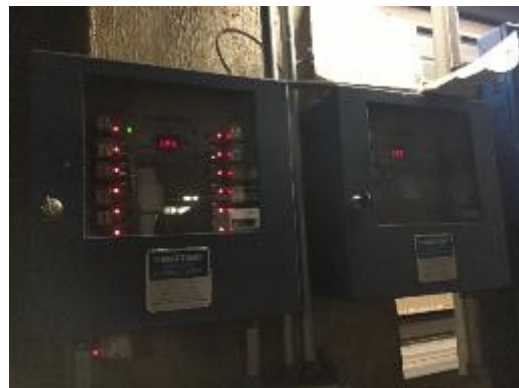
Heat Timer Boiler Controls
