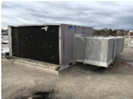
Roof Top Unit
