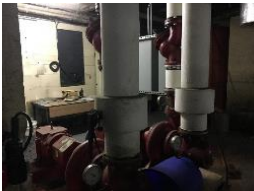
Hot Water Pumps and Motors
