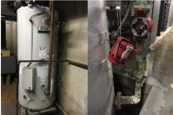
Inoperable Storage Tank Water Heater and Broken Hot water Pump Motor
