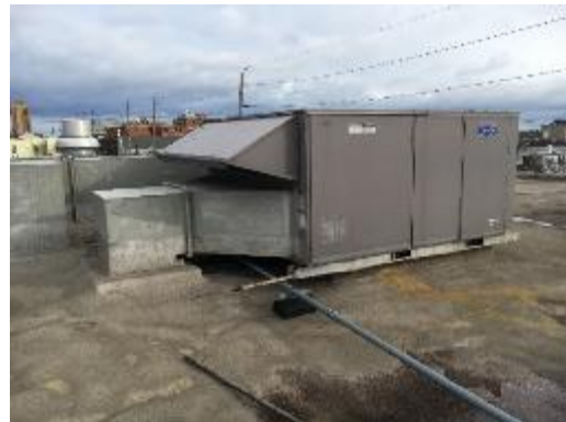
Roof Top Unit
