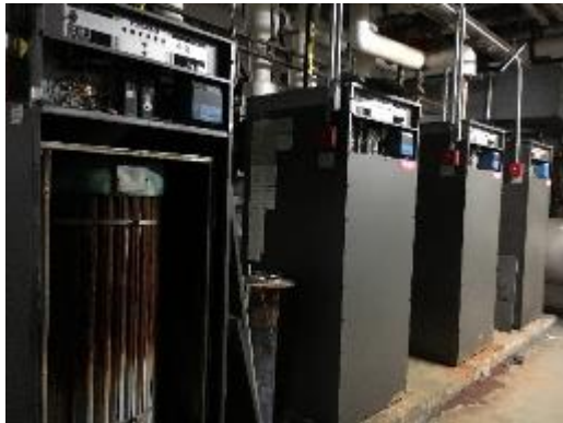
Hot Water Boilers
