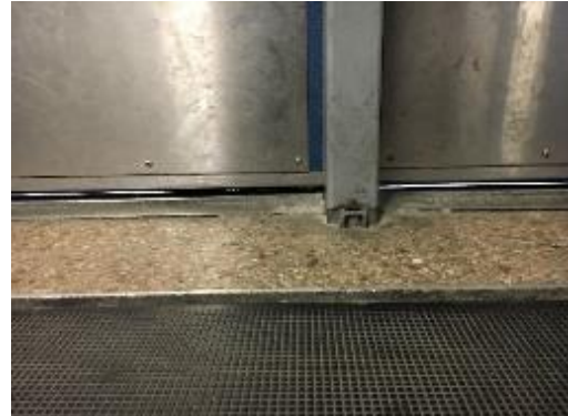
Weather-stripping in Poor Condition
