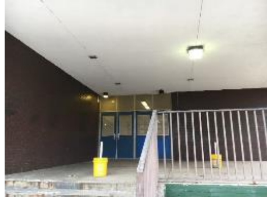
Surface Mounted HID Fixtures
