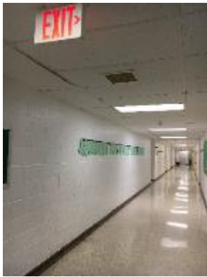
Linear T8 Troffer Fixtures and LED Exit Sign
