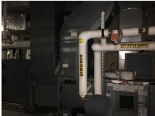
AHU with Hot Water Coil
