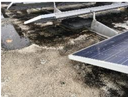
Roof in Poor Condition
