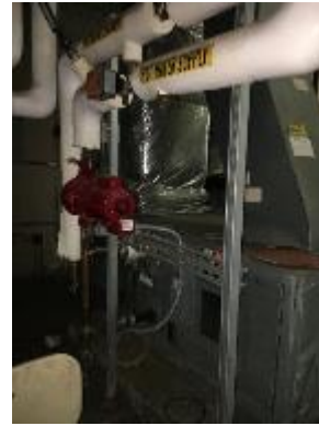
Hot Water Circulator Pump Motor for AHU
