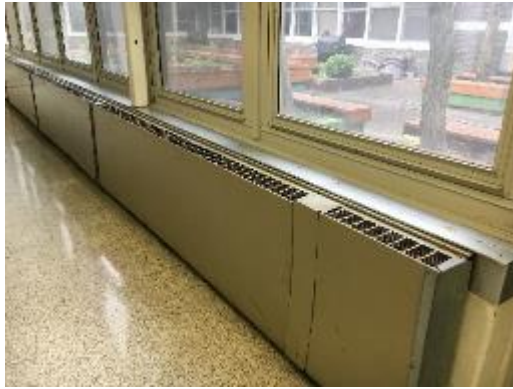
Perimeter Radiators in Hallway
