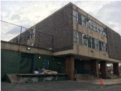
Various HID Fixtures
