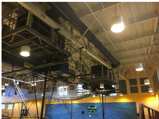
Main Gym Lighting
