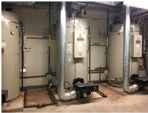
Custom Storage Tank Water Heaters
