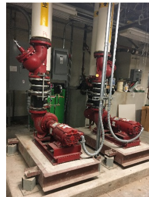
5 hp GSHP Loop Pumps
