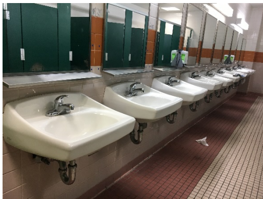
Restroom Hand Washing Sinks
