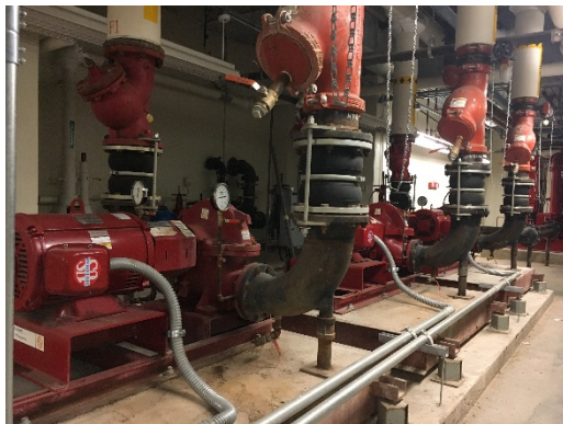
50 hp GSHP Loop Pumps
