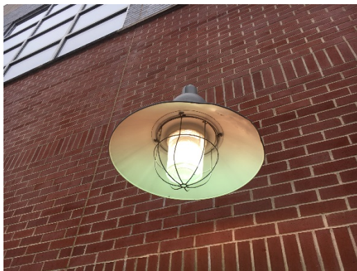
Wall Mounted Metal Halide Fixture
