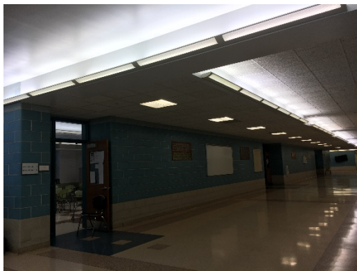
Hallway T8 Lighting
