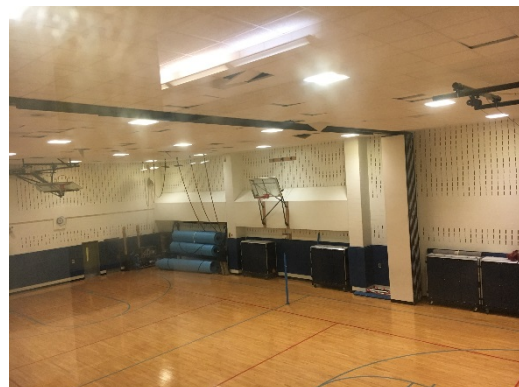
Auxiliary Gym Lighting
