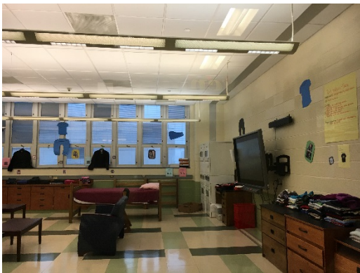
Linear Fluorescent T8 Fixtures
