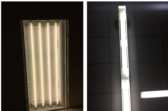
Linear Fluorescent T8 Fixtures
