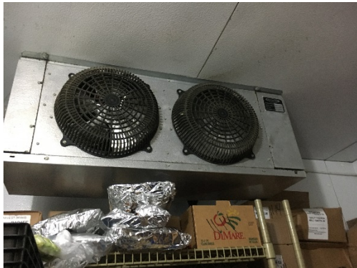
Walk-in Refrigeration Indoor Evaporator
