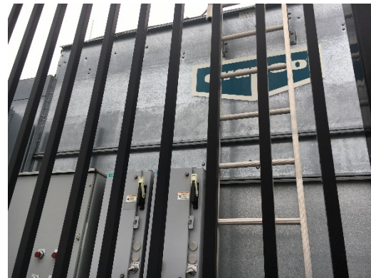
Evapco Cooling Tower
