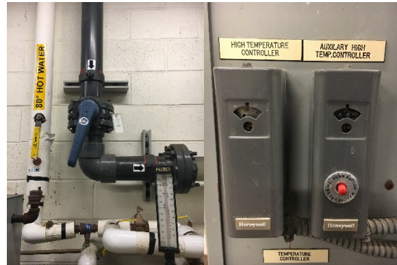
Piping and Temperature Gauges
