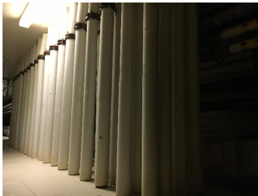
GSHP System Wells
