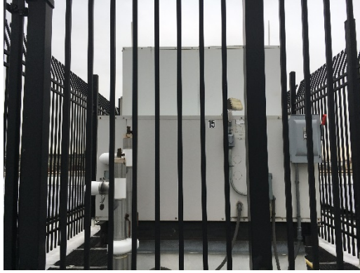
RTU with Gas Heat
