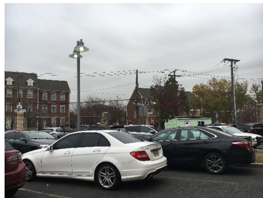
Pole Mounted Metal Halide Fixtures
