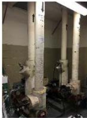
Hot Water Pumps and Motors
