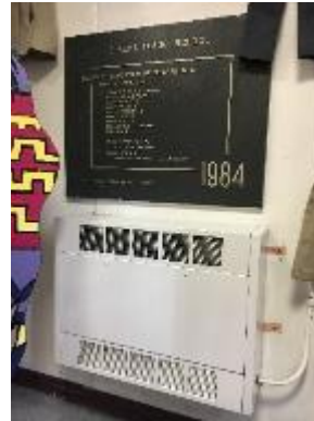
Electric Cabinet Unit Heater
