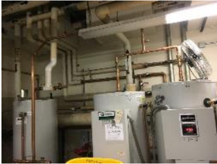
Domestic Hot Water Heaters and Storage Tanks
