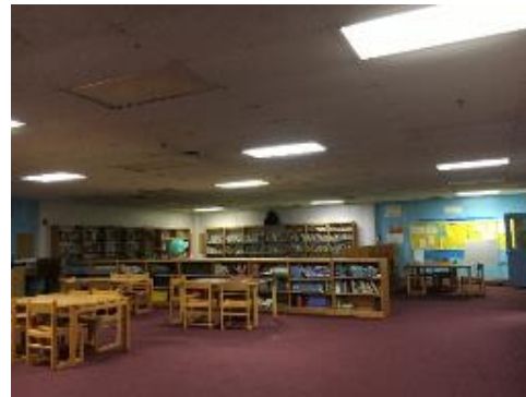
Recessed Troffer T8 Fixtures in Library
