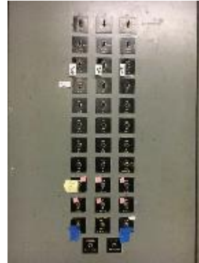
Manual HVAC Controls
