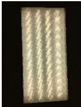
Recessed Troffer T8 Fixtures
