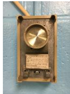
Thermostat in Poor Condition
