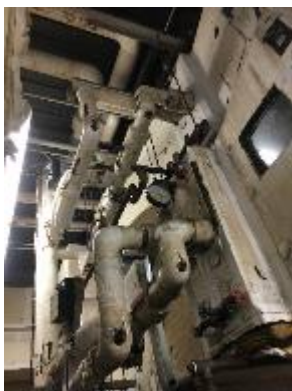
AHU with Chilled Water and Hot Water Coils
