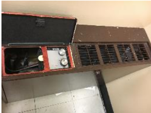
Electric Unit Heater
