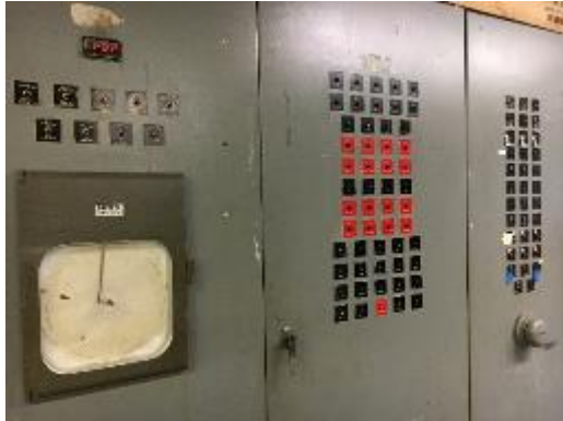
Manual HVAC Controls
