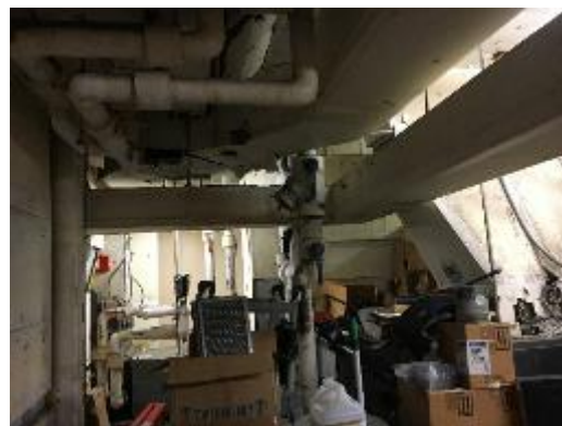
AHU with Chilled Water and Hot Water Coils
