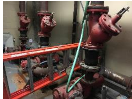
Condenser Water Pumps and Motors
