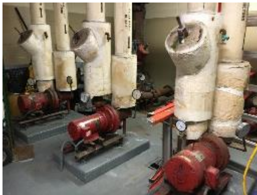
Chilled Water Pumps
