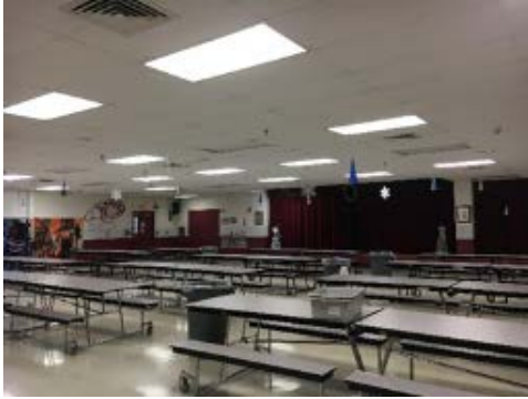
Recessed Troffer T8 Fixtures in Cafeteria
