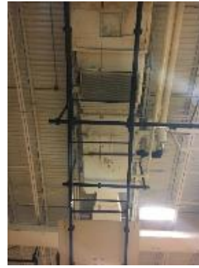
AHU in Gym
