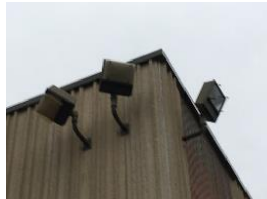
Wall-mounted HID Flood Fixtures
