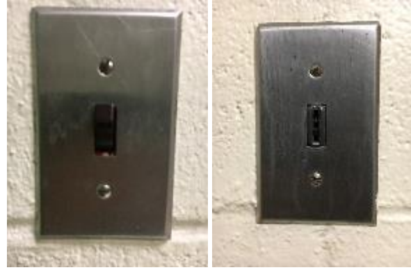
Wall Switch & Key Switch
