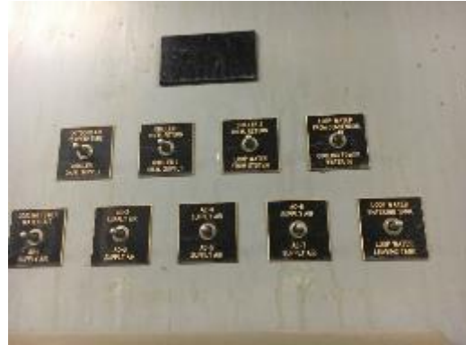
Manual HVAC Controls
