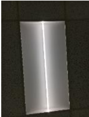
LED 2x4 Lay in Troffer Fixture
