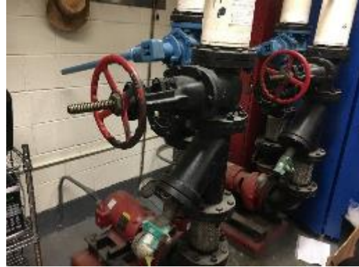
Heating Hot Water Pumps and Motors
