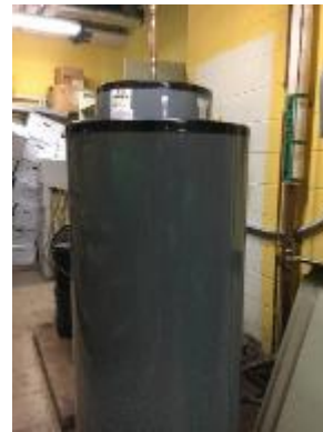
Domestic Water Heater in Mechanical Room
