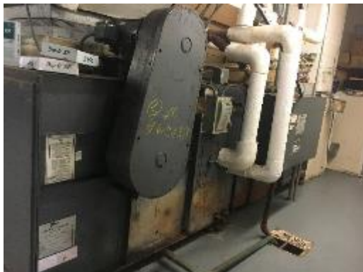
AHU in Mechanical Room
