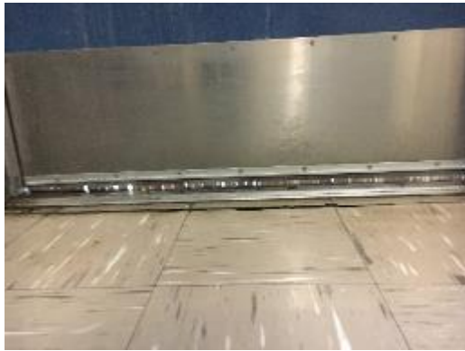
Exterior Door with Worn Weather-Stripping
