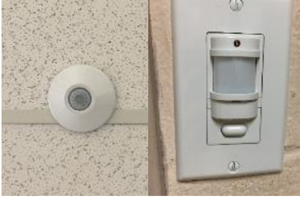
Ceiling-mounted & Wall Switch Occupancy Sensors
