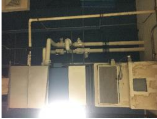
Shop/Storage Space AHU (Previously Gym)
