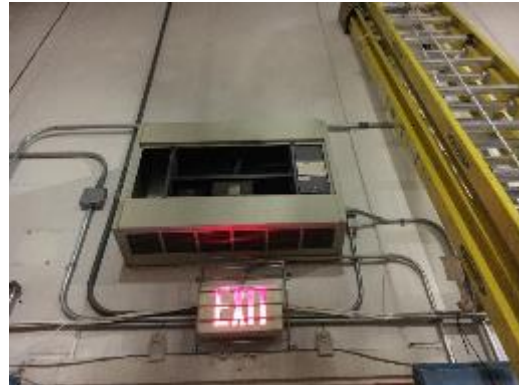
Electric Cabinet Unit Heater
