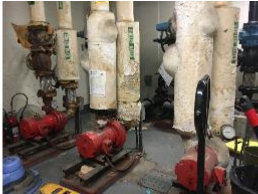
Chilled Water Pumps and Motors
