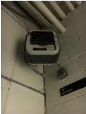
Electric Unit Heater
