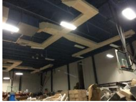
Shop/Storage Space AHU (Previously Gym)
