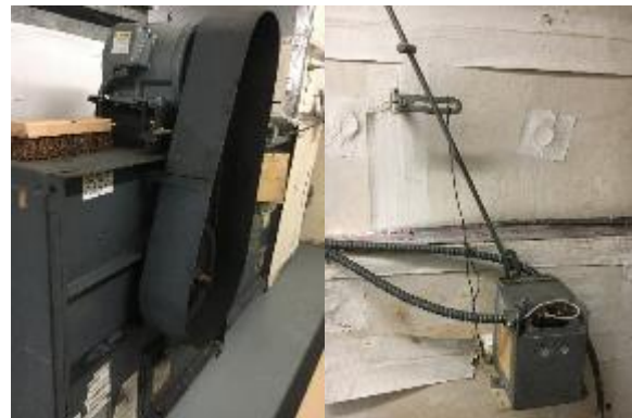
AHU in Mechanical Room
