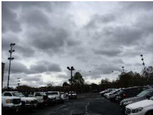
Pole-mounted HID Fixtures
