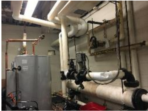
Heat Exchanger for Domestic Hot Water
