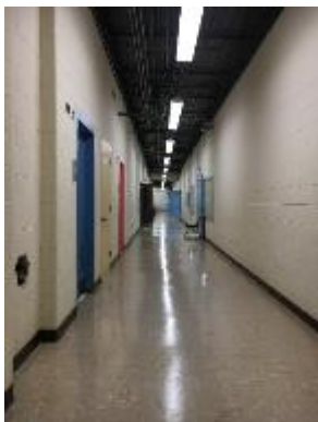
Linear Fluorescent T8 Unistrut Mounted Fixtures
