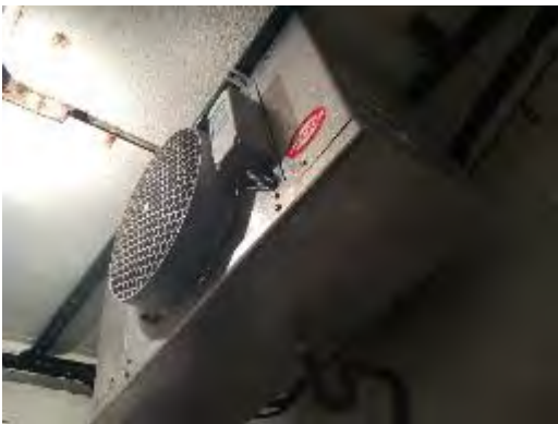
Walk-in Cooler Evaporator
