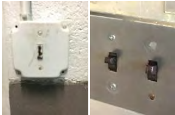
Key Switch and Wall Switches
