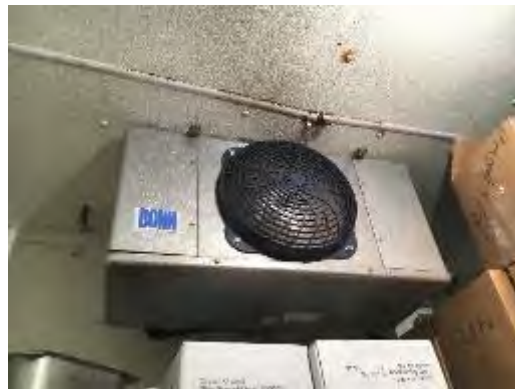
Walk-in Cooler Evaporator
