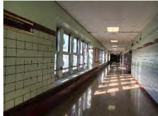
Linear Fluorescent T8 Recessed Troffer Fixtures
