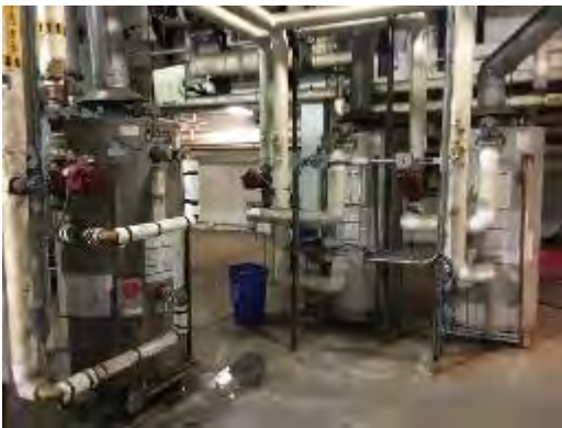
Domestic Storage Tank Water Heaters
