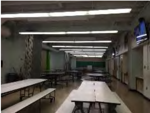
Linear Fluorescent T8 Wrap Fixtures
