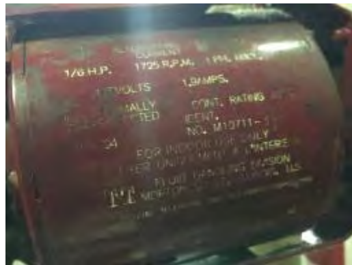
Circulation Pump Motor
