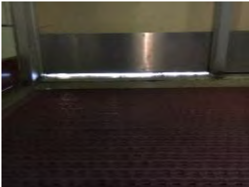
Door with Missing Weather Stripping
