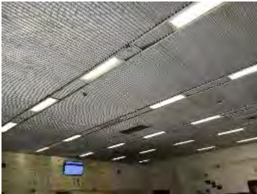
Linear Fluorescent T8 Fixtures in Cafeteria
