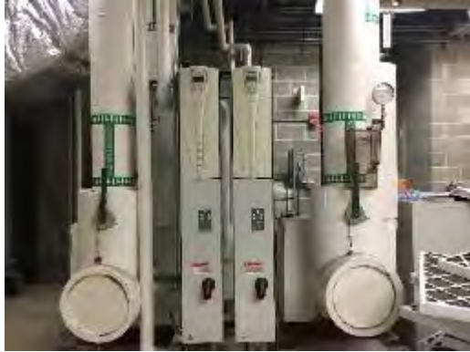
Ground Source Water Pumps and VFDs
