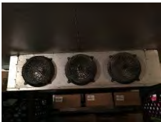
Walk-in Cooler Evaporator
