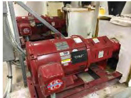
Hot Water Pump Motors
