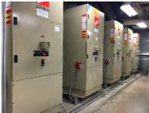
Hot Water Boilers
