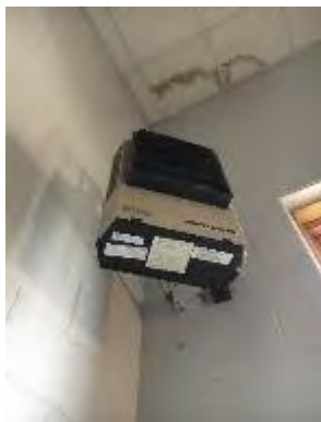
Electric Unit Heater
