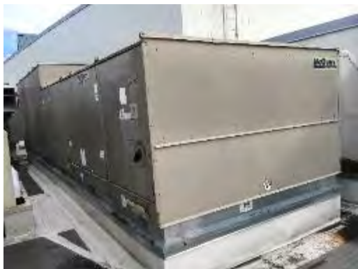
Roof Top Unit
