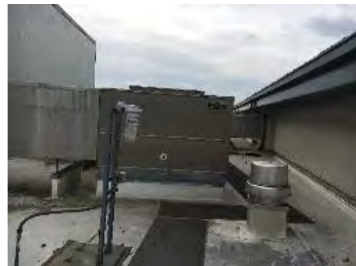
Roof Top Unit
