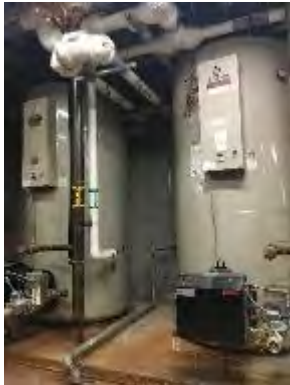
Old Custom Gas Water Heaters—No Longer in Use
