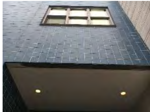
CFL Recessed Can Fixtures
