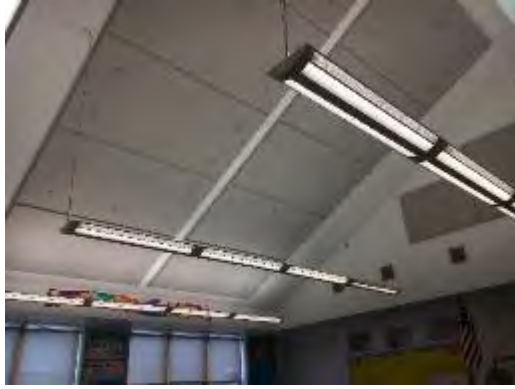
Linear Fluorescent T8 Pendant-mounted Fixtures
