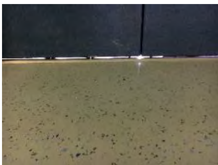
Door with Worn Weather-Stripping
