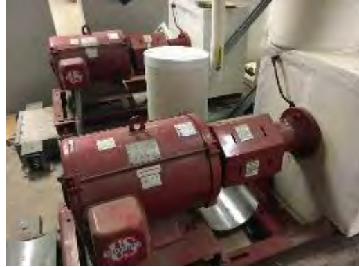
Ground Source Water Pump Motors
