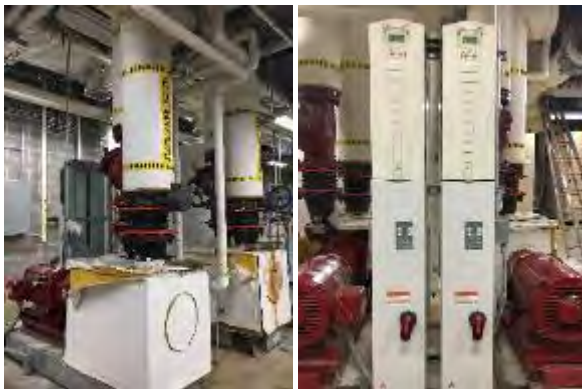
Hot Water Pumps and VFDs
