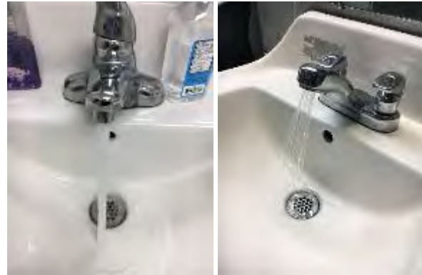
High-flow Sink Aerator vs Low-flow Sink Aerator
