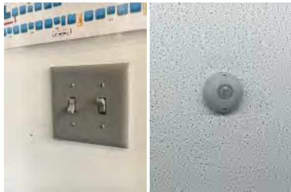
Wall Switches and Occupancy Sensor
