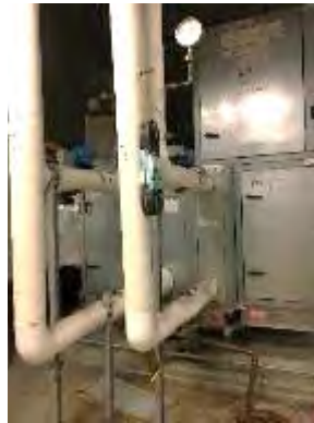
Make Up Air Unit
