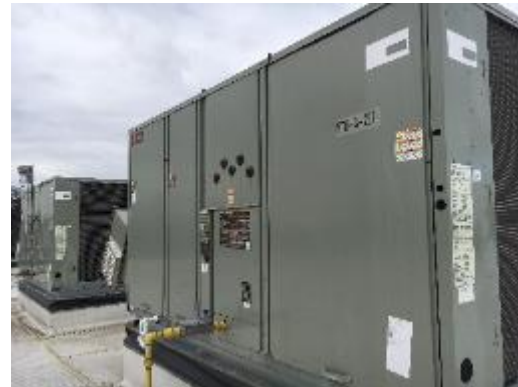
Roof Top Units
