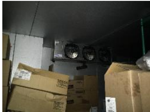
Walk-in Freezer Evaporator
