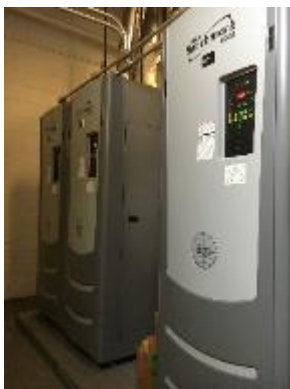
Hot Water Boilers
