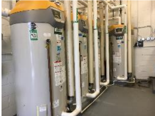
Storage Tank Water Heaters
