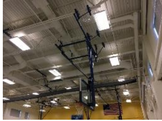
T8 High Bay Lighting in Gym
