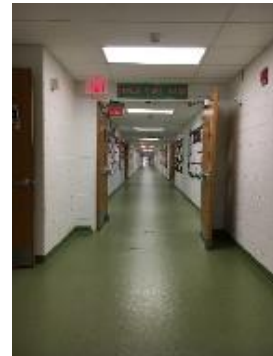
Linear Fluorescent T8 Troffer Fixtures
