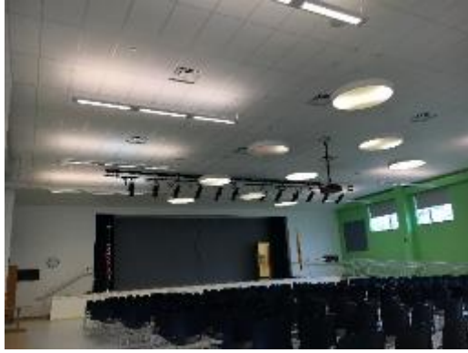
T8 Pendant-mounted Lighting
