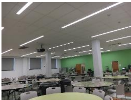
LED Strip Fixtures in Cafeteria
