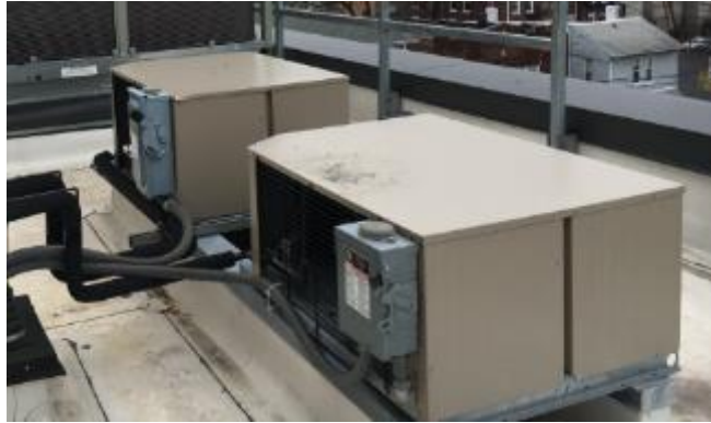
Outdoor Compressors for Walk-in Refrigeration Equipment
