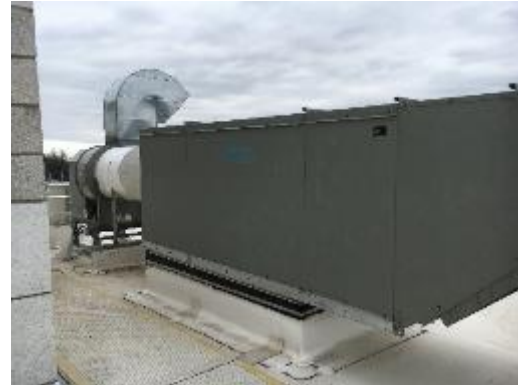
Make Up Air Unit
