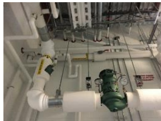
Hot Water Pump and Motor
