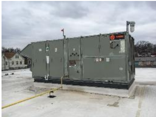
Roof Top Unit
