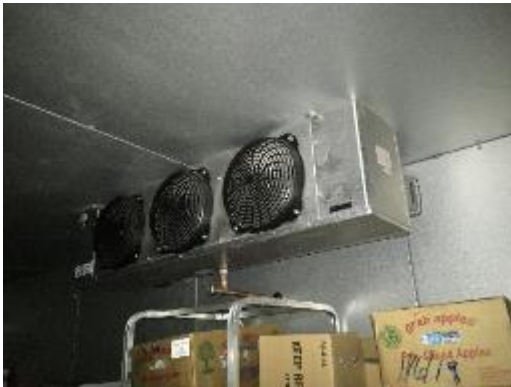
Walk-in Cooler Evaporator
