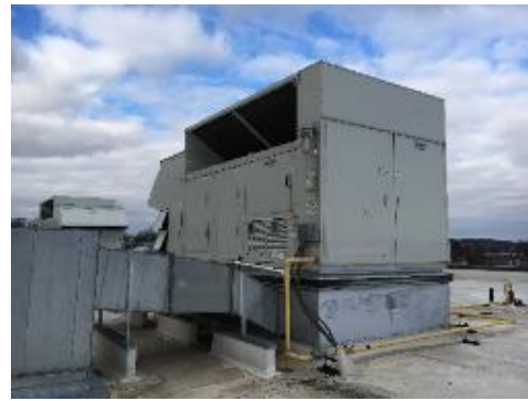
Energy Recovery Units
