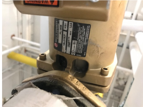
DHW Circulation pump
