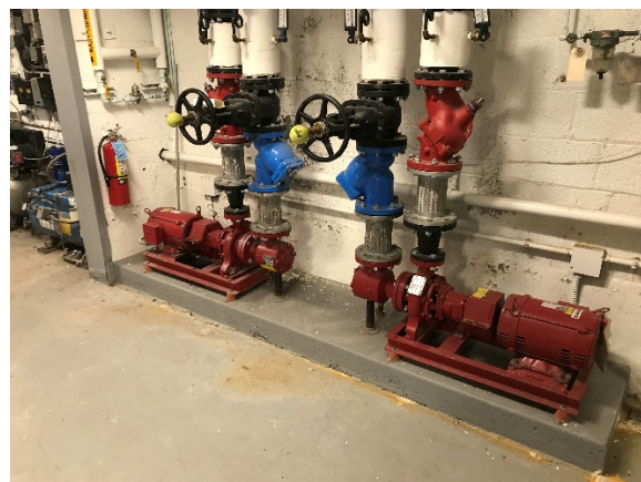
Heating hot water pumps
