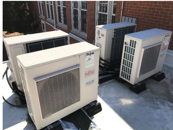
Condensing Units on roof
