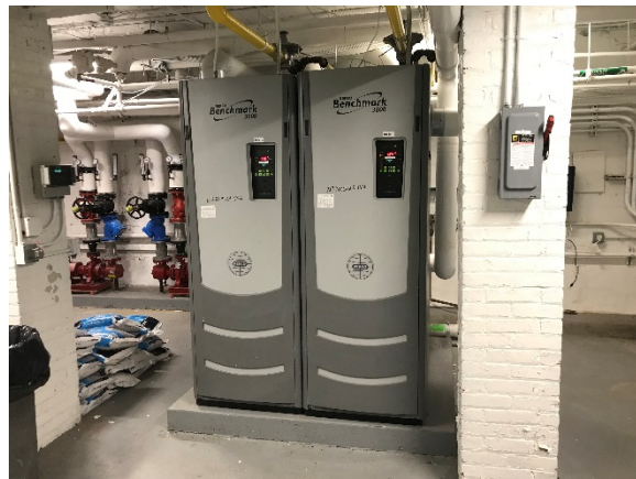
Hot water boilers
