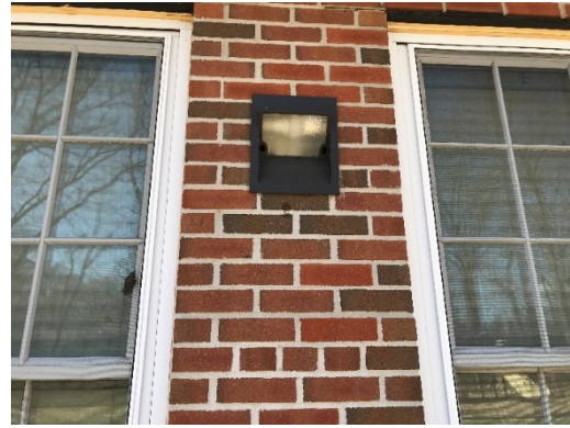
Flushed mounted wall fixture
