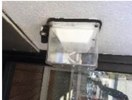
Exterior Lighting Fixture
