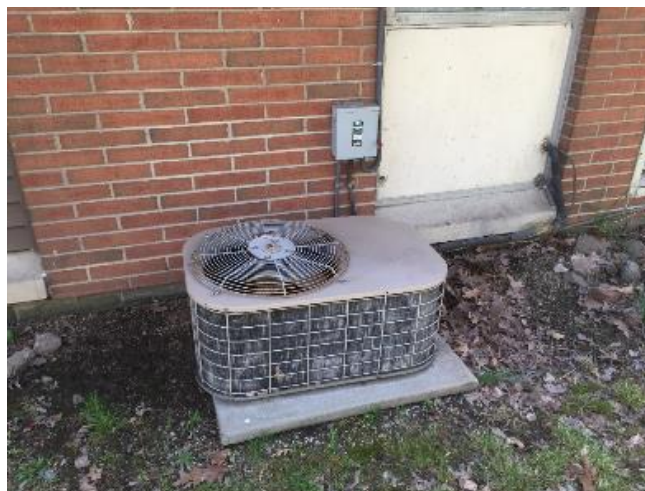
Split AC Unit
