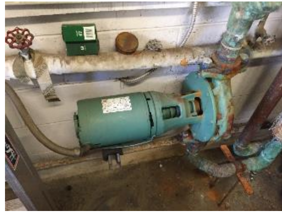
Heating Hot Water Pump
