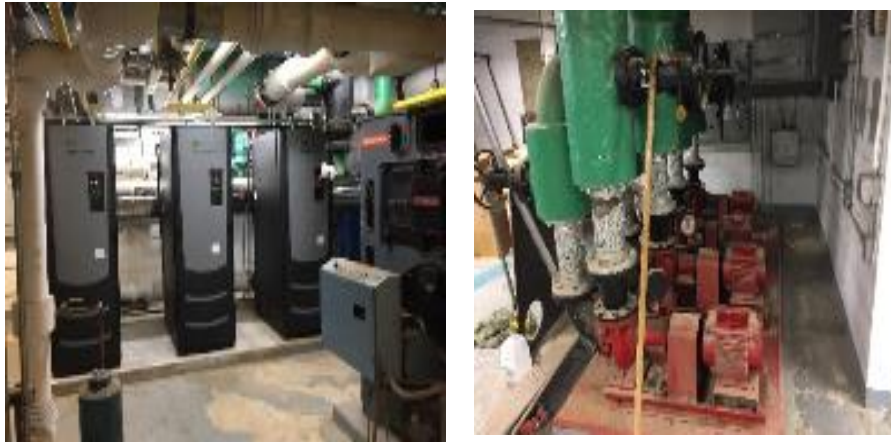
Figure 10 – Heating Hot Water Equipment
