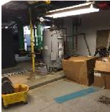
Figure 12 – Domestic Hot Water Equipment
