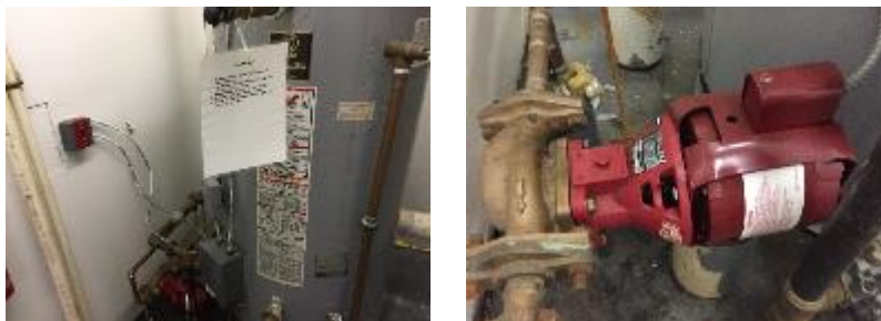
Figure 11 – Domestic Hot Water Equipment
