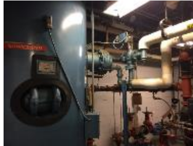
Figure 12 – Domestic Hot Water Equipment
