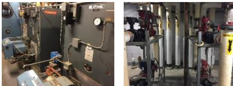
Figure 10 – Heating Hot Water Equipment
