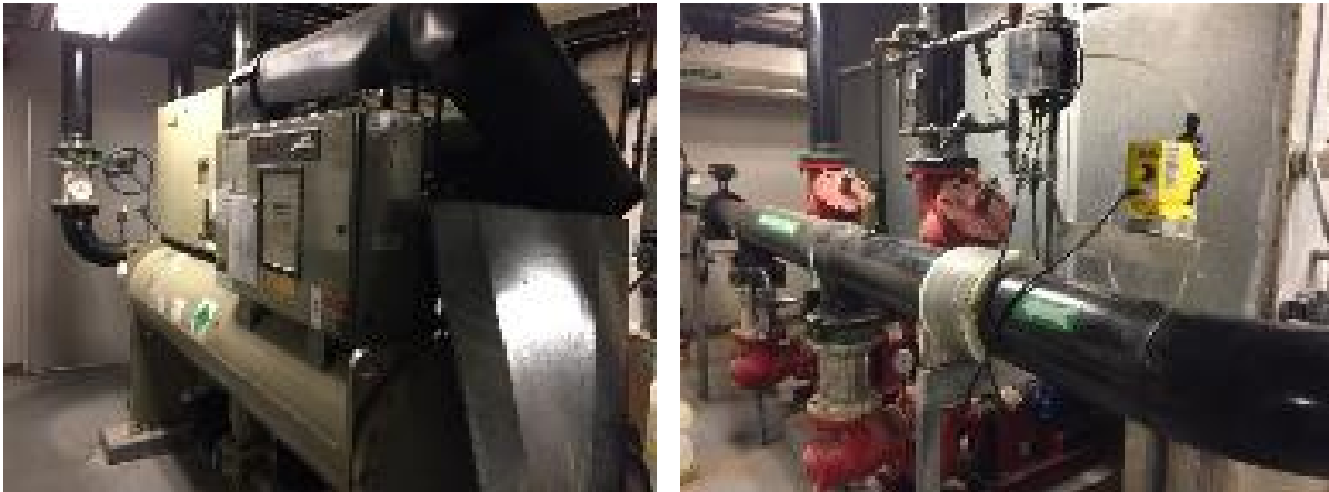
Figure 9 – Chilled and Condenser Water Equipment
