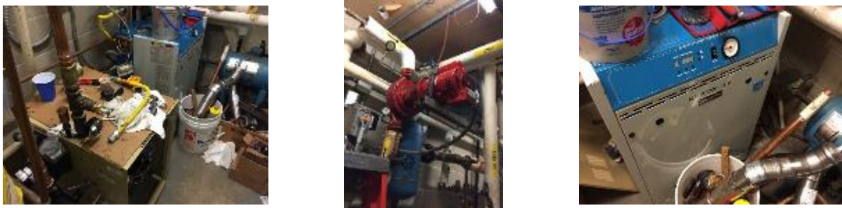
Figure 8 – Heating Hot Water Equipment
