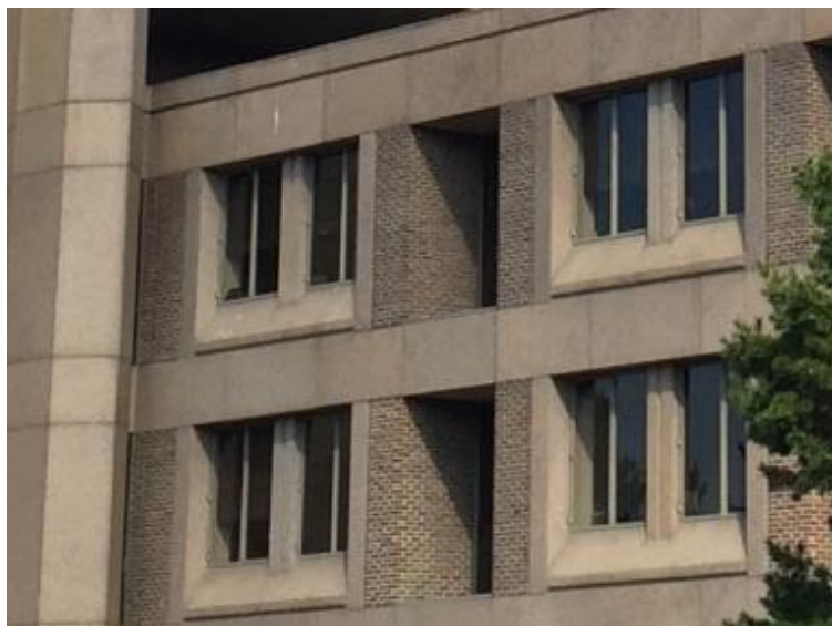
Exterior Walls & Windows
