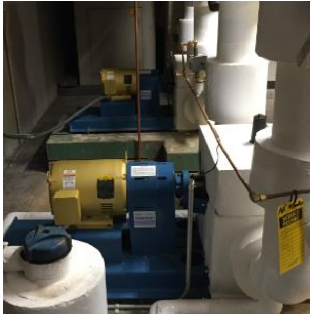
Chilled Water Pumps
