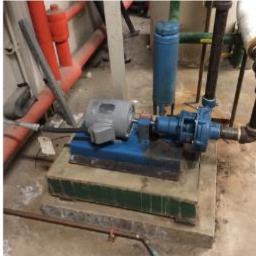
Heating Hot Water Pump
