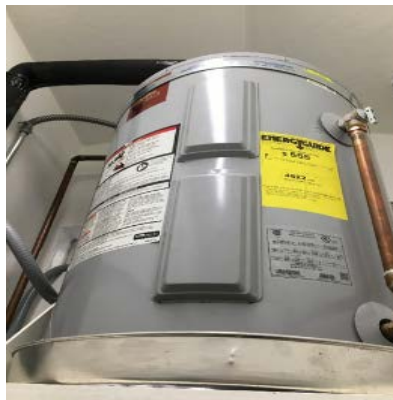
Domestic Water Heater
