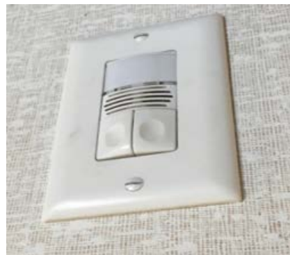
LED Lamp & Wall Mounted Occupancy Sensor
