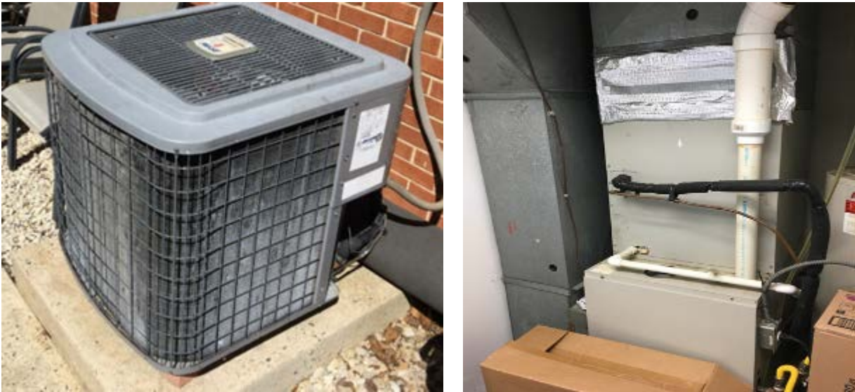
Cooling and Heating System
