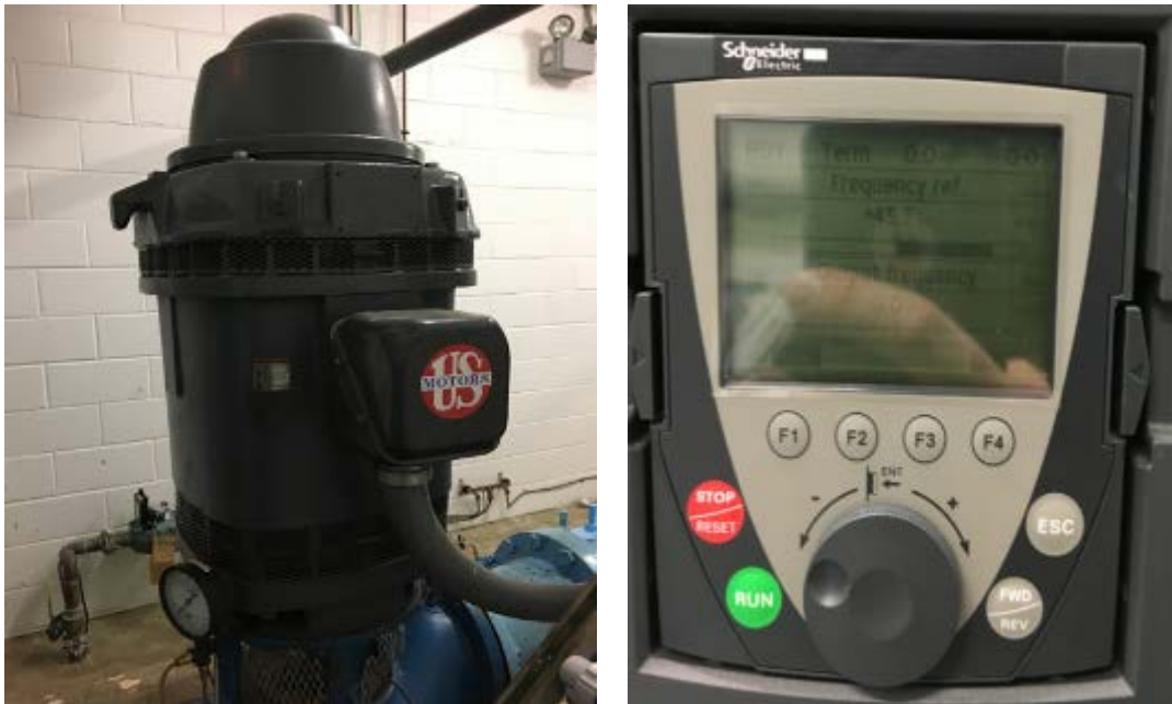
Well #9 Pump & VFD
