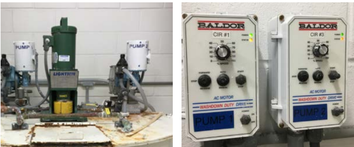
Two Lime Pumps & Mixing Pump
