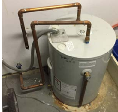
Image 5: 19-Gallon, Electric Water Heater
