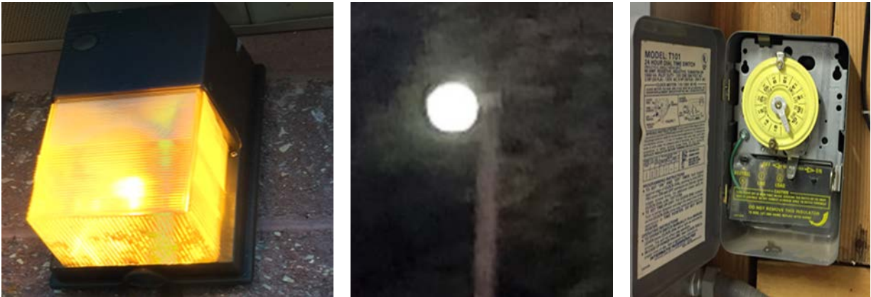
Image 3: Exterior Lighting Systems
