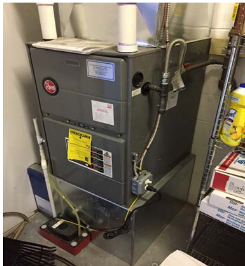
Image 4: Rheem Gas-Fired Furnace
