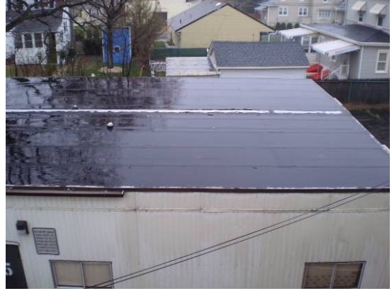
Rubber membrane roof of modular
