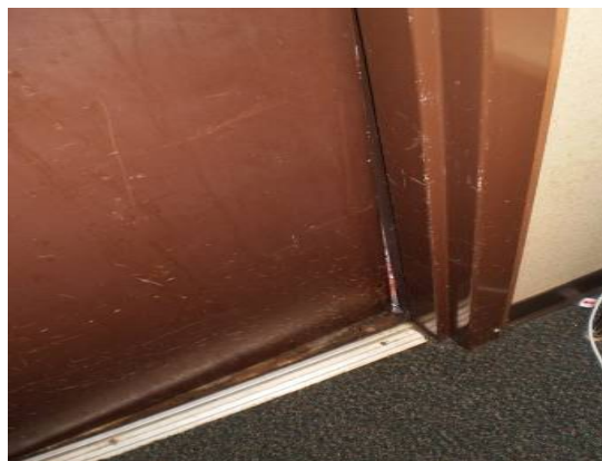
Exterior door in Modular classroom
