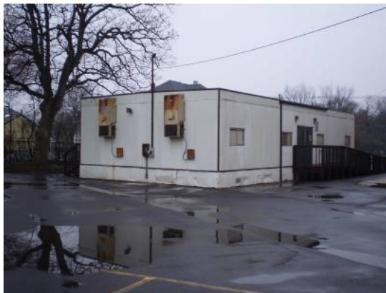
Modular classroom building
