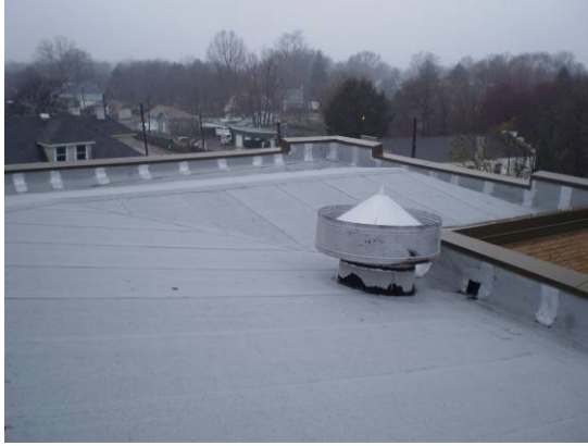
Asphalt roof of school
