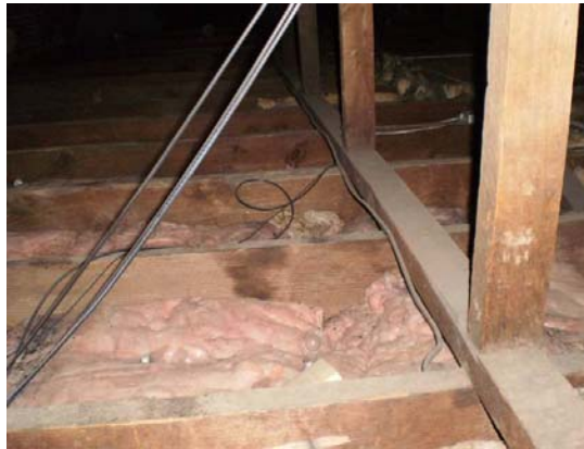
Attic above classroom #7
