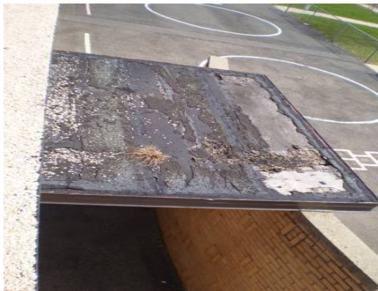
Roof above School Entrance
