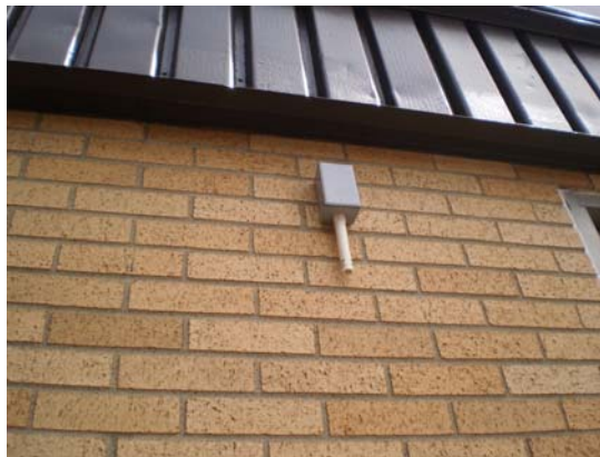
Brick veneer on exterior wall
